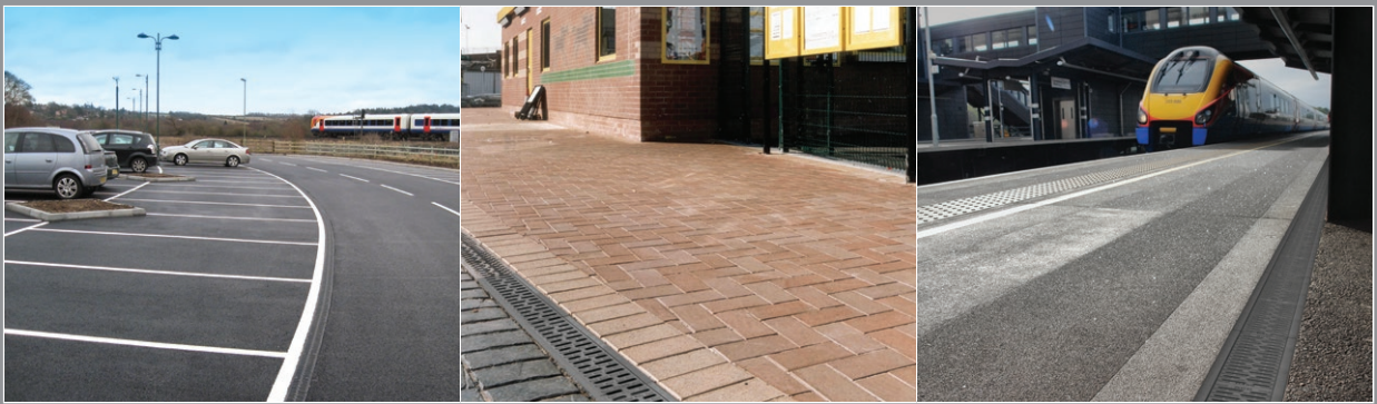
Black - Asphalt installations
