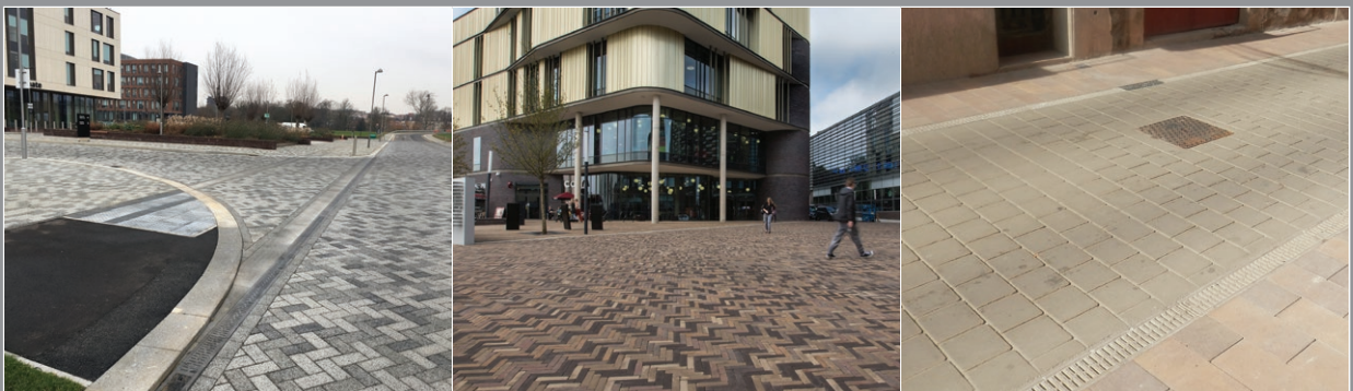
Natural - Paving installations
