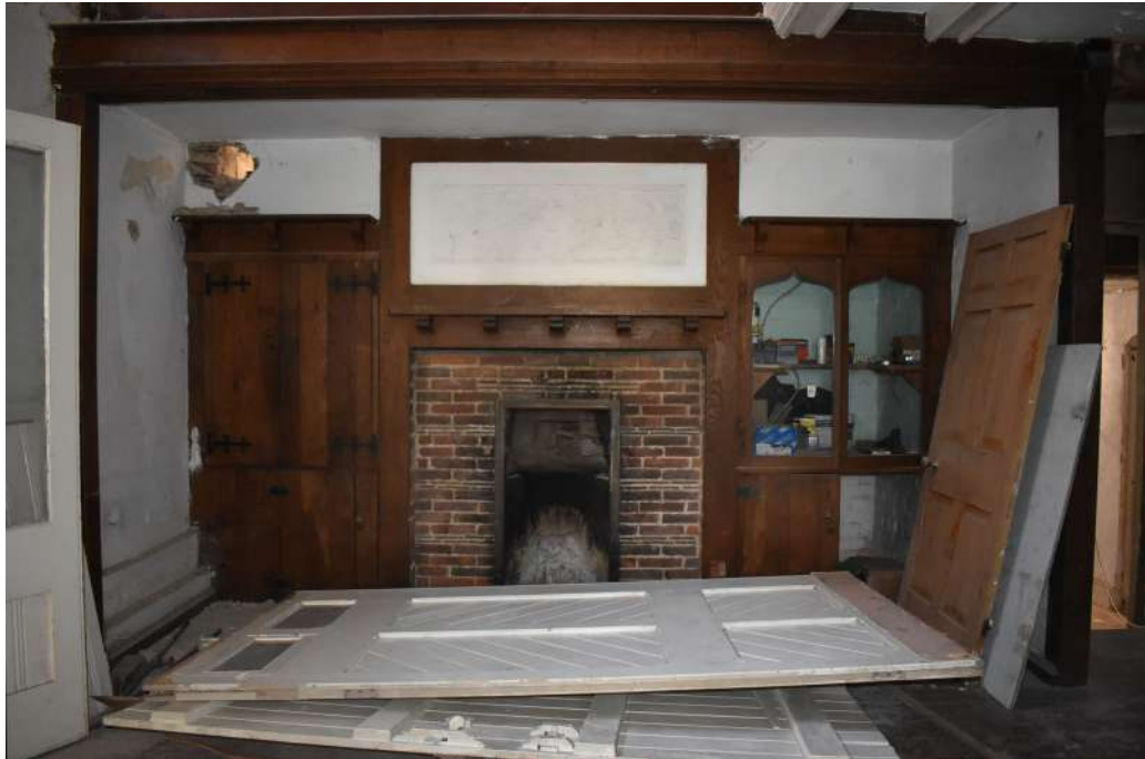
Photograph 28 Detail of fireplace in room 8. Photograph taken facing north-east.
