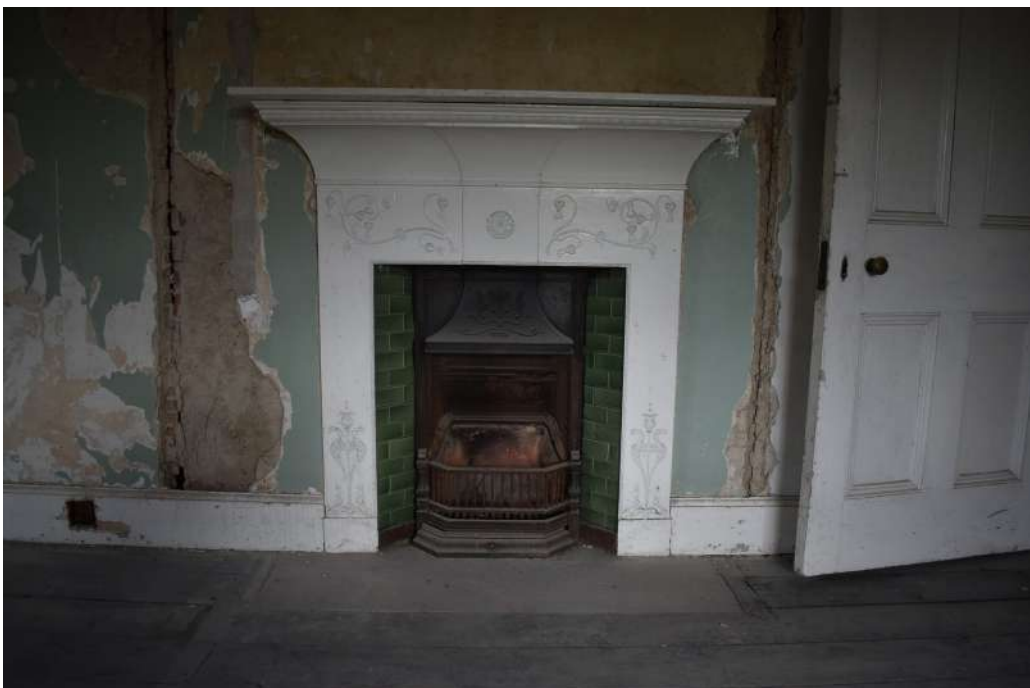
Photograph 39 Detail of fireplace in room 16. Photograph taken facing north-east.
