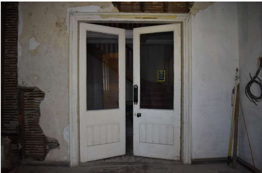
Photograph 21 Detail of doors in room 2. Photograph taken facing south-east.
