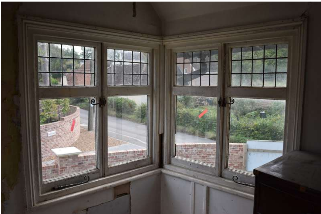
Photograph 51 Detail of window in room 26. Photograph taken facing south.
