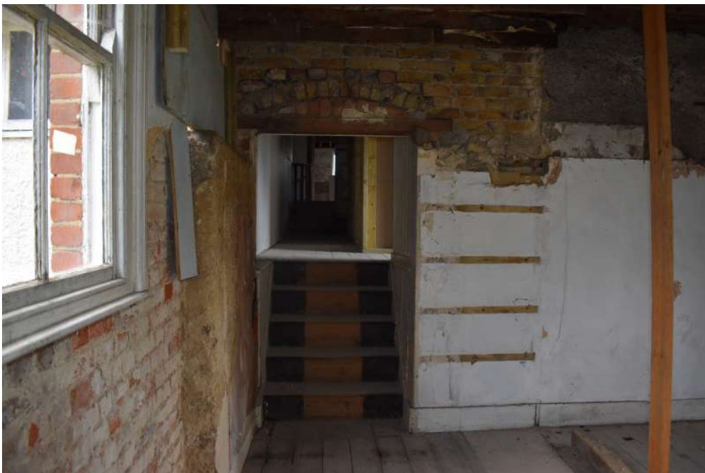
Photograph 43 Detail of opening in room 18. Photograph taken facing south-west.
