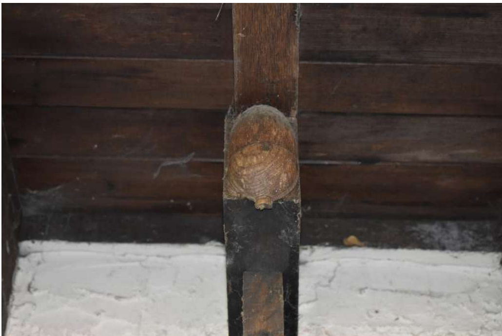
Photograph 8 Detail of carved acorn in doorway of north-west elevation. Photograph taken facing south-east.
