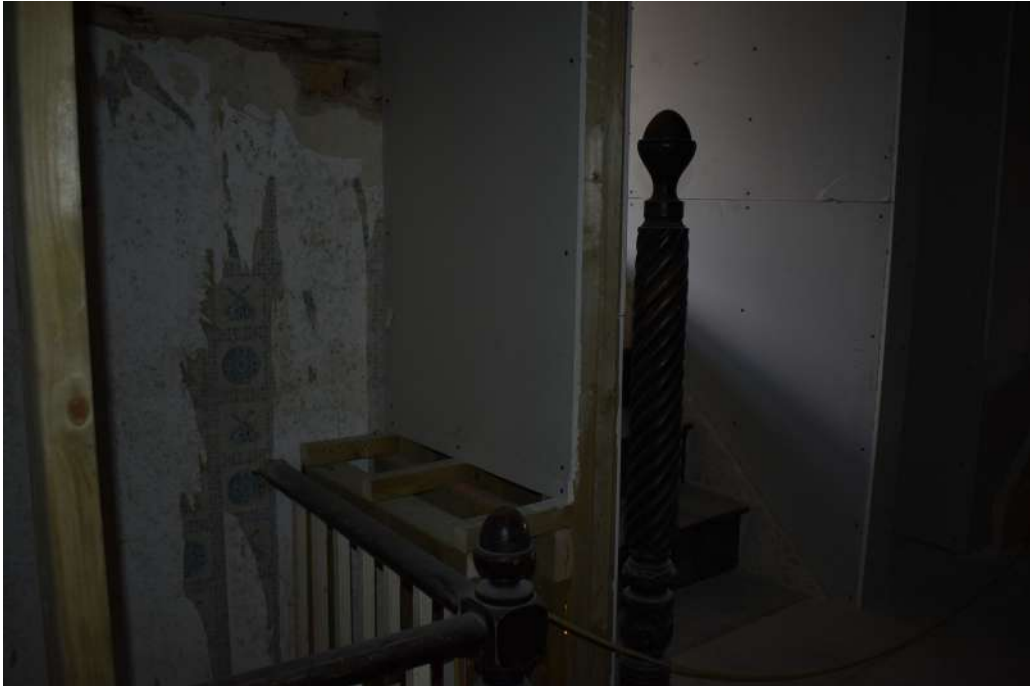
Photograph 50 Detail of newel posts in room 23. Photograph taken facing south.
