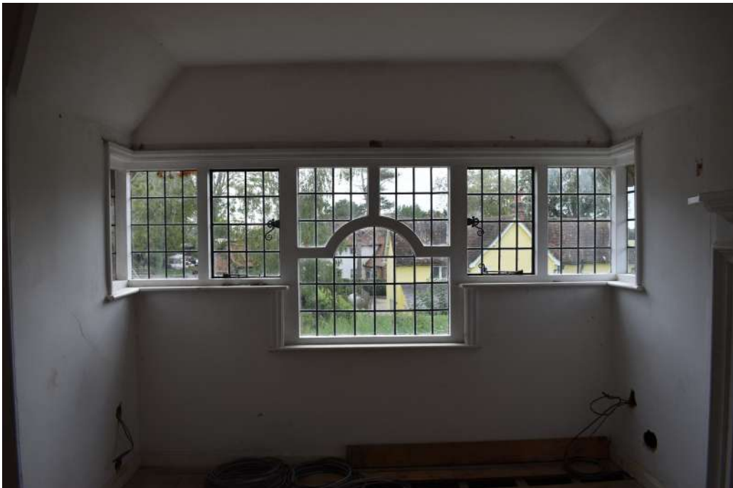
Photograph 37 Detail of window in room 14. Photograph taken facing north-west.
