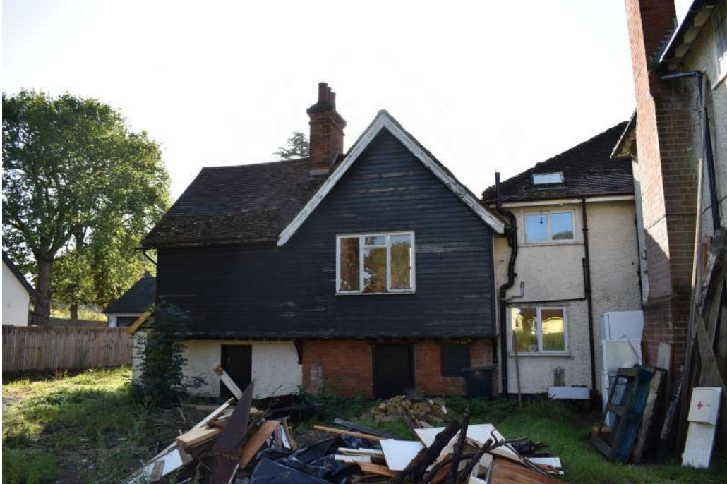
Photograph 9 North-west elevation. Photograph taken facing south-east.
