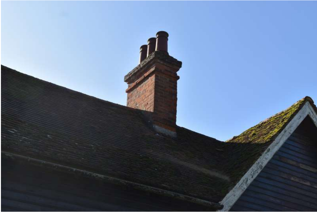
Photograph 4 Detail of north-eastern chimney. Photograph taken facing south.
