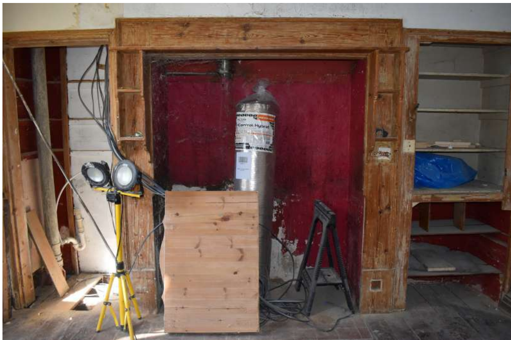
Photograph 29 Detail of fireplace in room 9. Photograph taken facing north-west.
