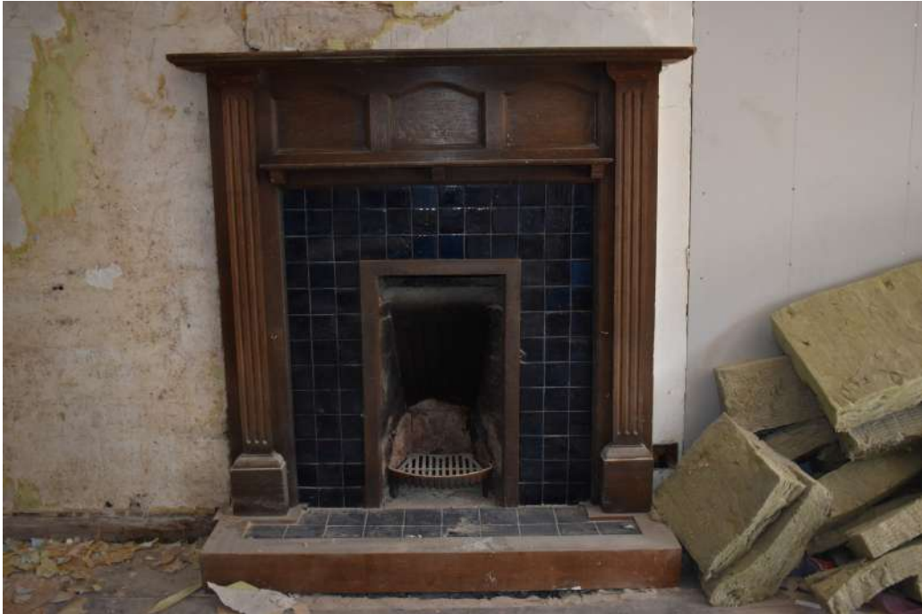
Photograph 52 Detail of fireplace in room 26. Photograph taken facing north-east.
