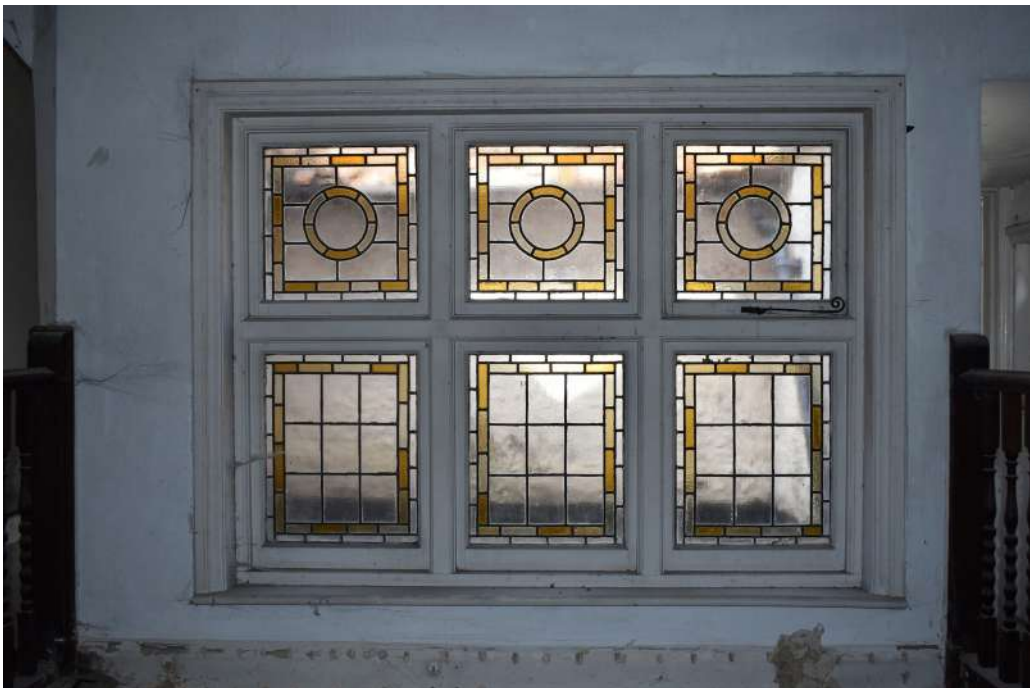
Photograph 47 Detail of window in room 21. Photograph taken facing north-west.
