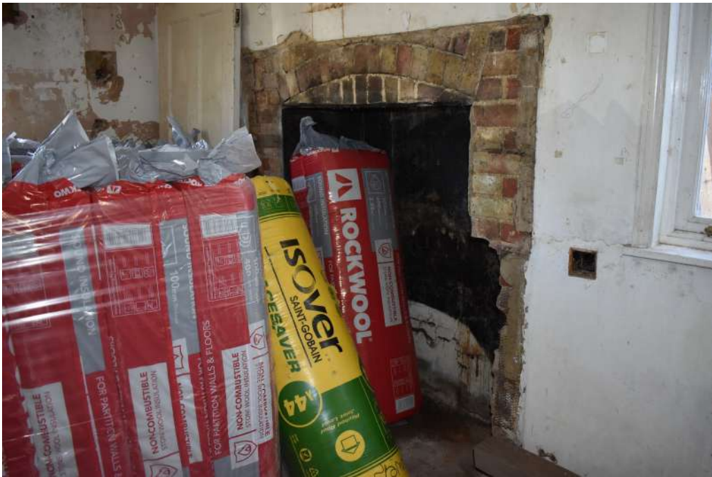
Photograph 19 Detail of fireplace in room 1. Photograph taken facing north.
