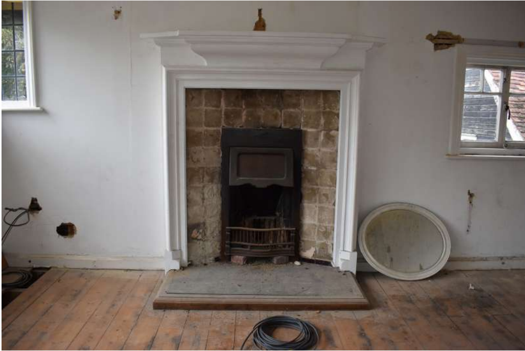
Photograph 38 Detail of fireplace in room 14. Photograph taken facing north-east.
