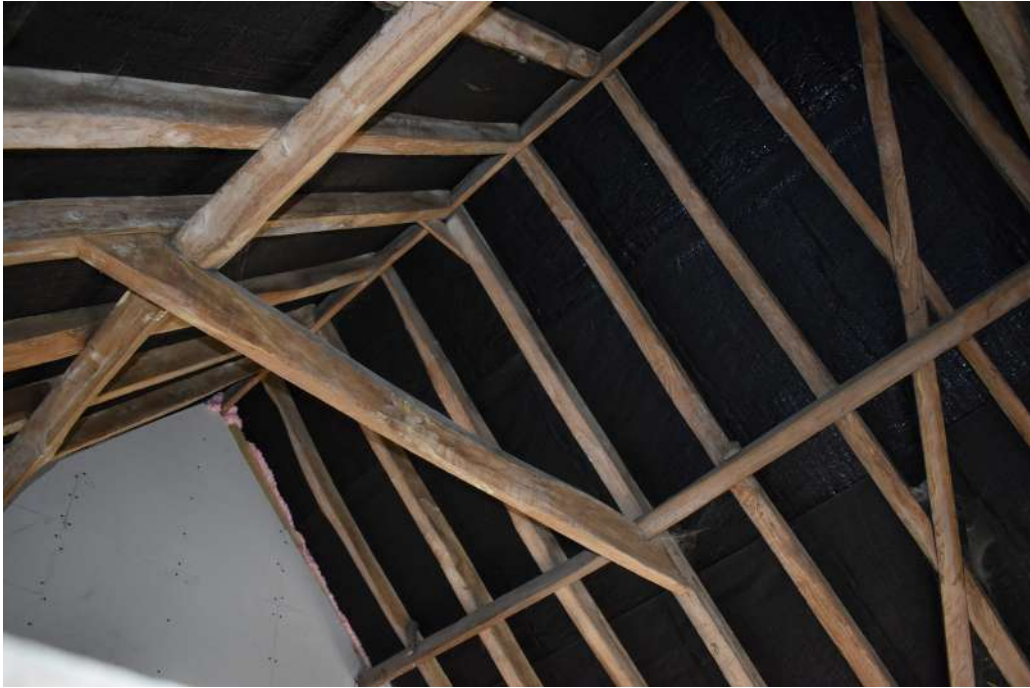
Photograph 16 Detail of roof structure above room 22. Photograph taken facing south-east.
