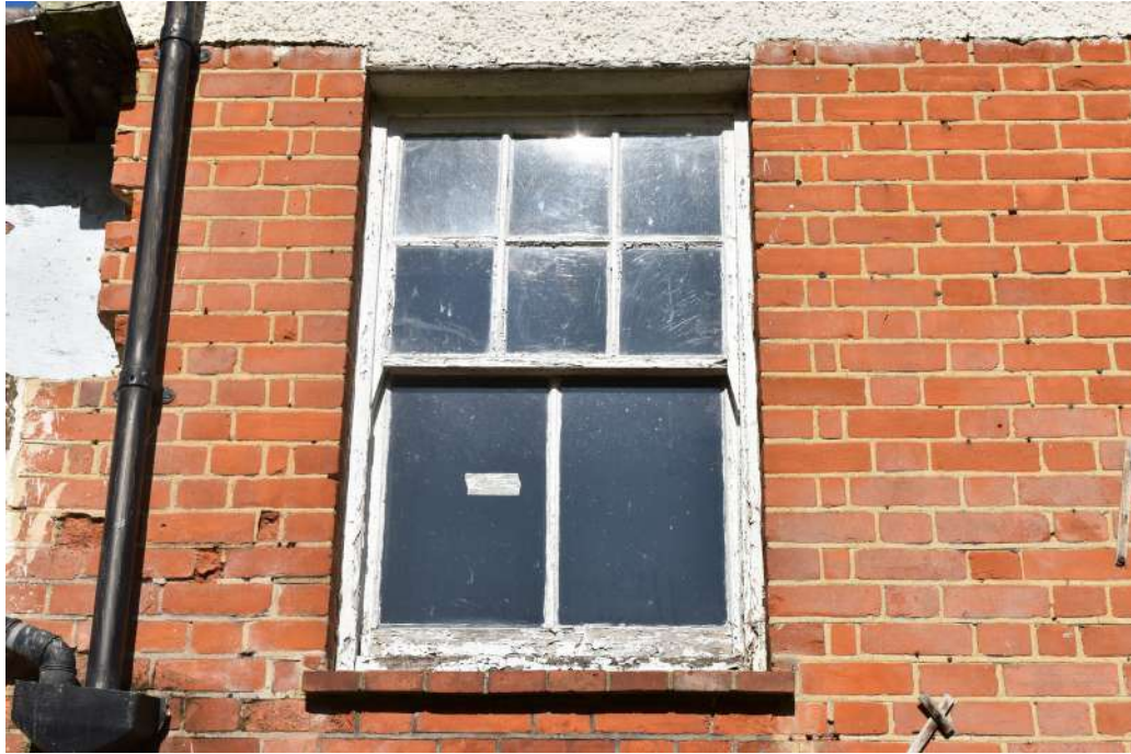
Photograph 13 Detail of window on south-east elevation. Photograph taken facing north-west.
