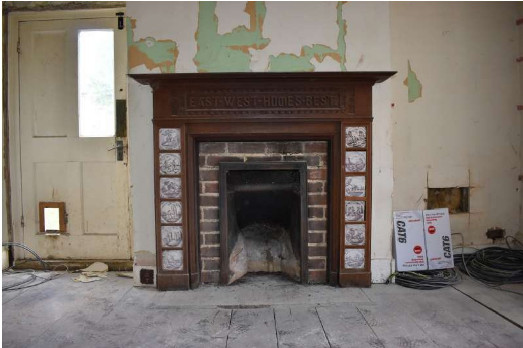
Photograph 36 Detail of fireplace in room 13. Photograph taken facing south-east.
