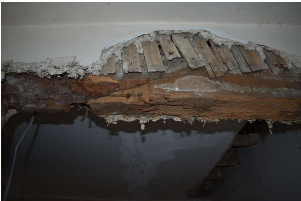
Photograph 35 Detail of splayed scarf-joint in girthing-beam in room 13. Photograph taken facing north-west.
