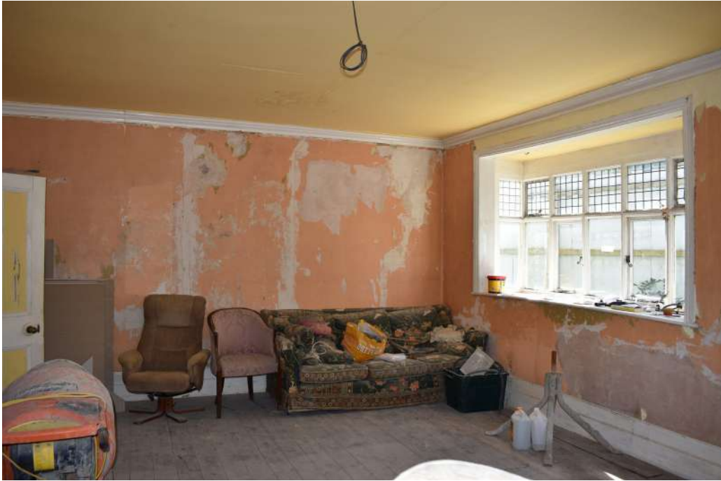
Photograph 22 Interior of room 3. Photograph taken facing south.
