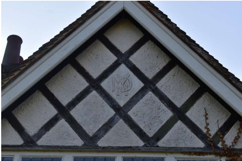
Photograph 6 Detail of monogram emblem and exposed timber-framing on north-west elevation. Photograph taken facing south-east.
