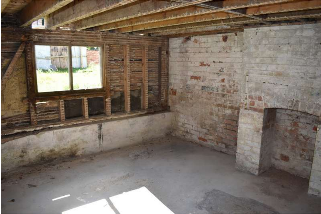
Photograph 24 Interior of room 5. Photograph taken facing south.
