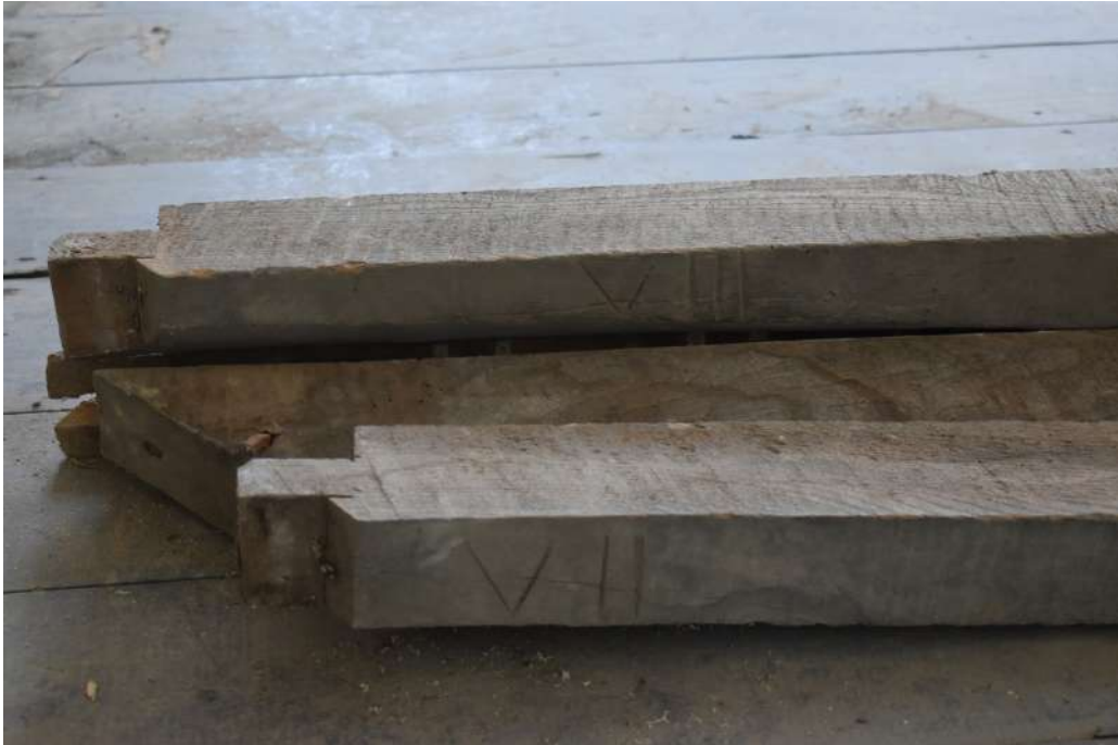
Photograph 40 Detail of carpenter's marks on loose timbers in room 16.
