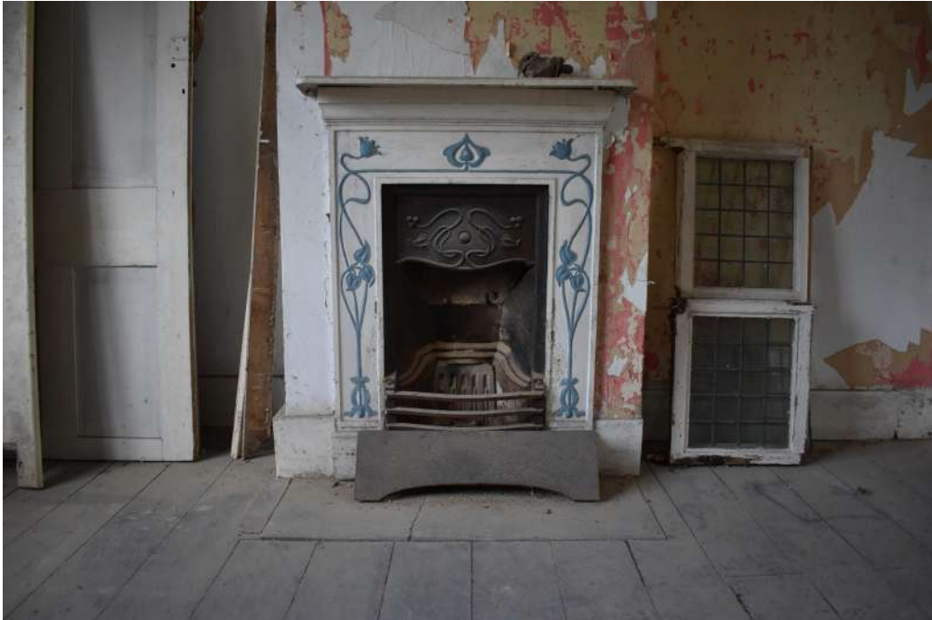
Photograph 44 Detail of fireplace in room 18. Photograph taken facing north-east.
