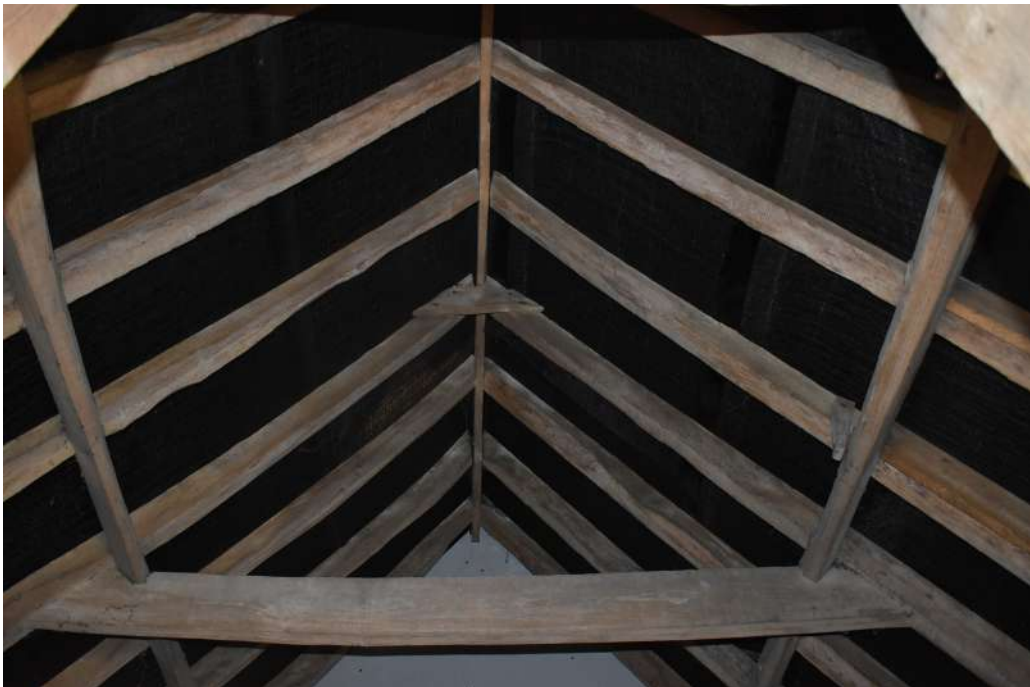
Photograph 17 Detail of roof structure above room 24. Photograph taken facing north-west.
