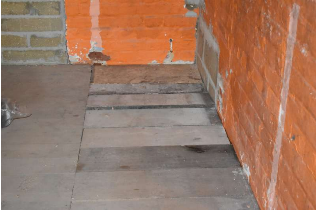
Photograph 26 Detail of blocked cellar entrance. Photograph taken facing south.
