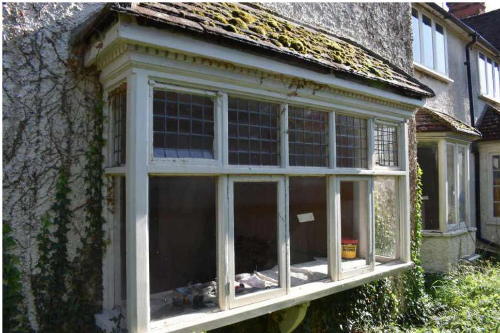
Photograph 14 Detail of window on south-west elevation. Photograph taken facing north.
