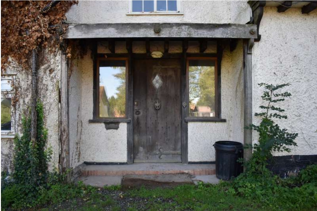
Photograph 7 Detail of door on north-west elevation. Photograph taken facing south-east.
