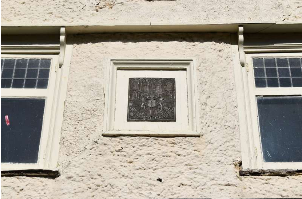
Photograph 12 Detail of sundial on south-east elevation. Photograph taken facing north-west.
