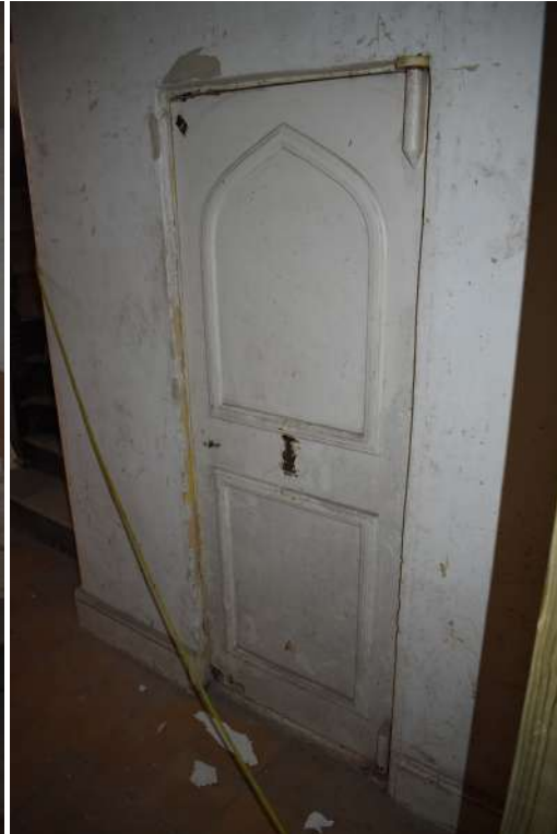
Photograph 31 Detail of safe in room 10. Photograph taken facing east.
