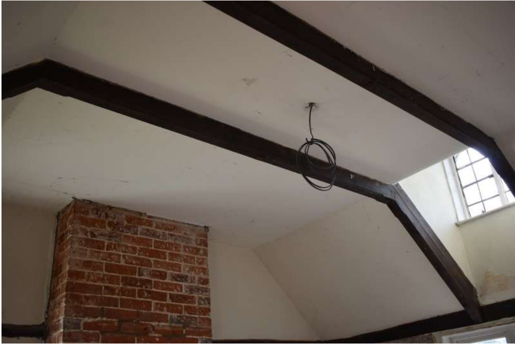
Photograph 54 Detail of exposed roof structure in room 27. Photograph taken facing south.
