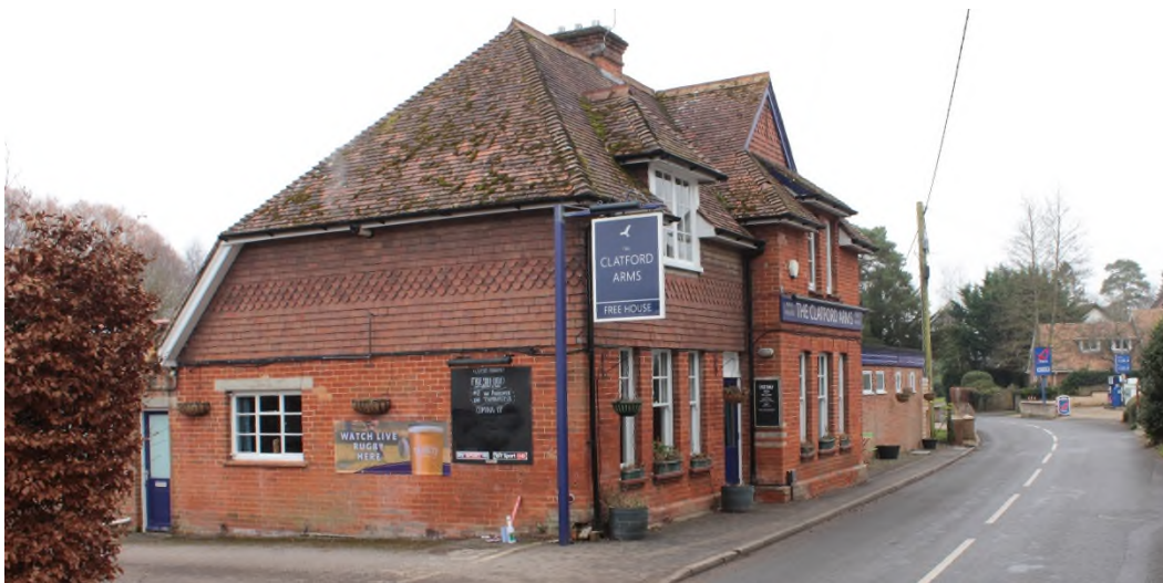
Figure 3 The Clatford Arms, front and north elevations.
