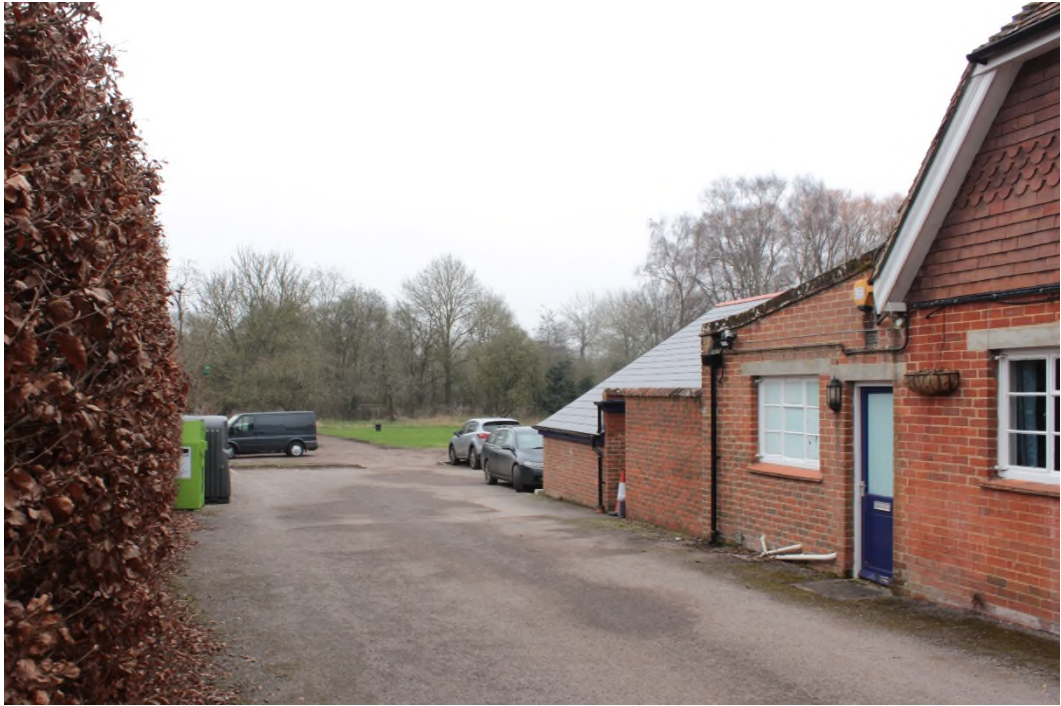
Figure 5 The view into the plot to the rear of the Clatford Arms from the Longstock Road.
