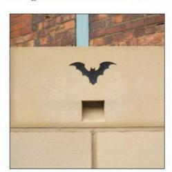
The Forticrete Bat Box has been developed to be used in new build construction or renovation where there is a requirement to provide a habitat for pipistrelle bats.
