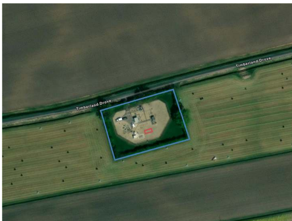
Figure 1: Image showing the proposed site and the wider site owned by Cadent Gas.
