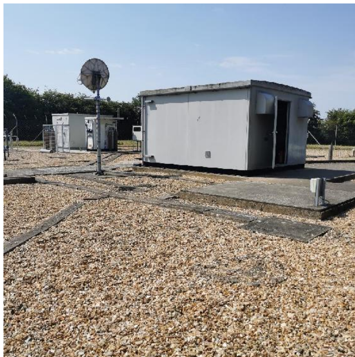
Photograph 12 – Buildings on the application site
