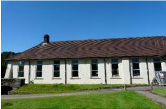
Zone A where the works will commence.
