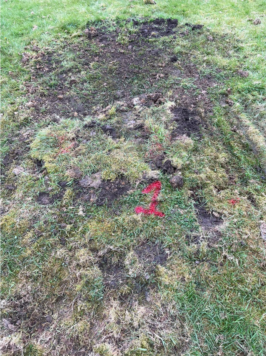
Figure 6 - Test pit remediation
