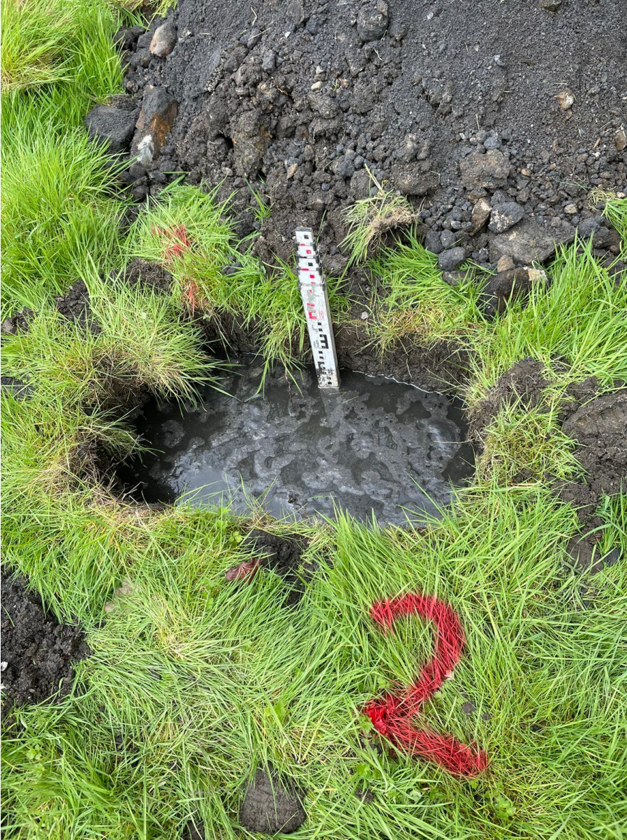
Figure 4 – TP2 after filling
