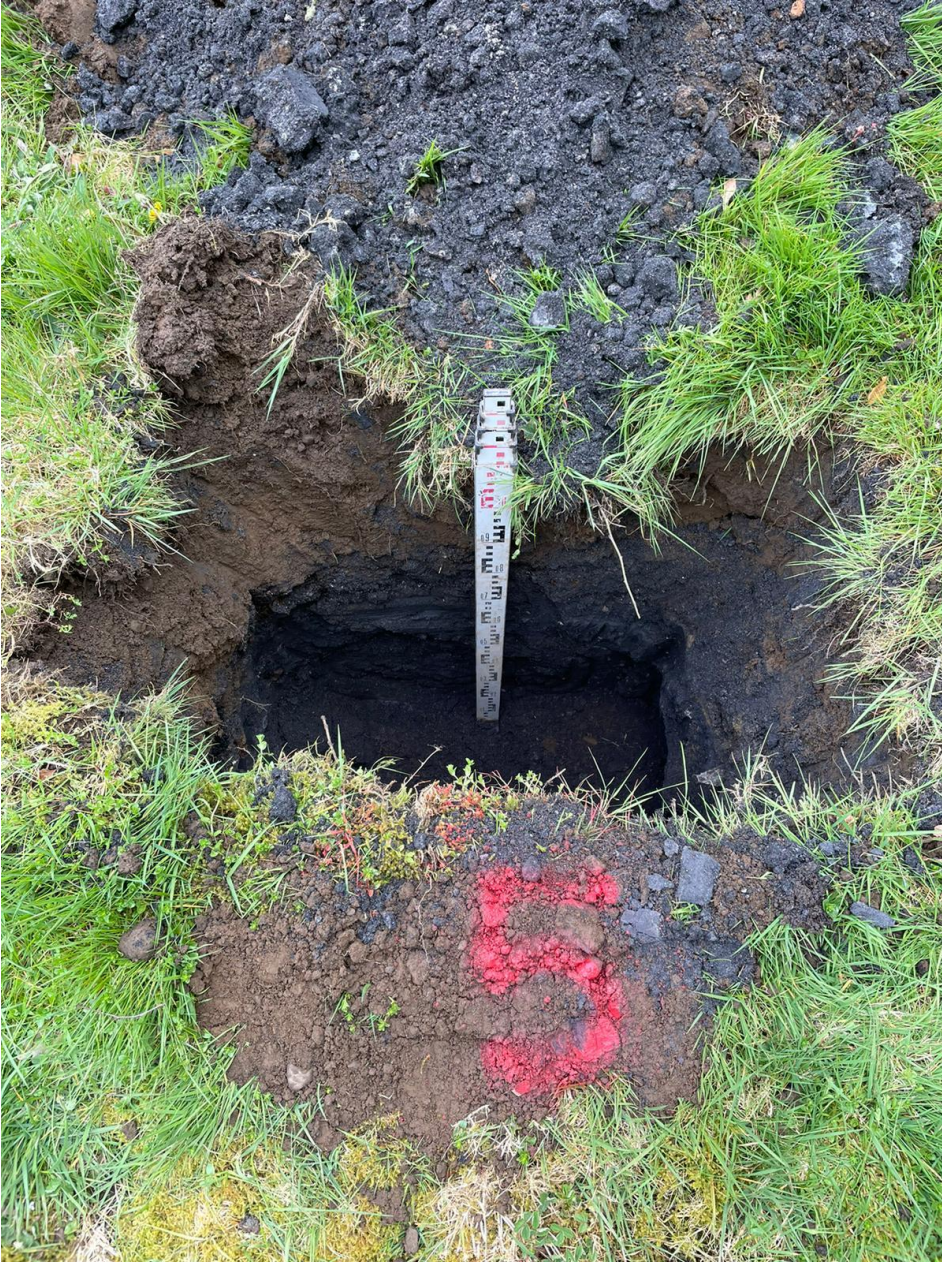
Figure 5 - TP5 after excavation
