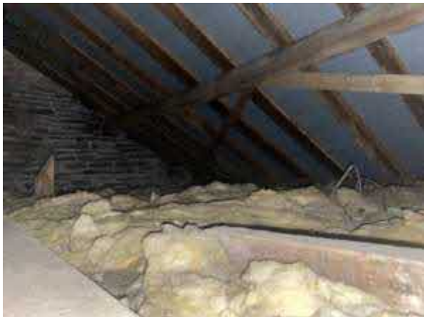
Photo 23: Fiberglass Insulation Present Inside the Void – B1
