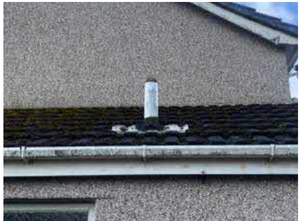
Photo 24: Vent with Lead Flashing at the Base – B1
