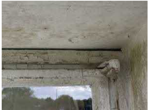
Photo 18: Gap Present Surrounding Metal Window Fixtures – B1
