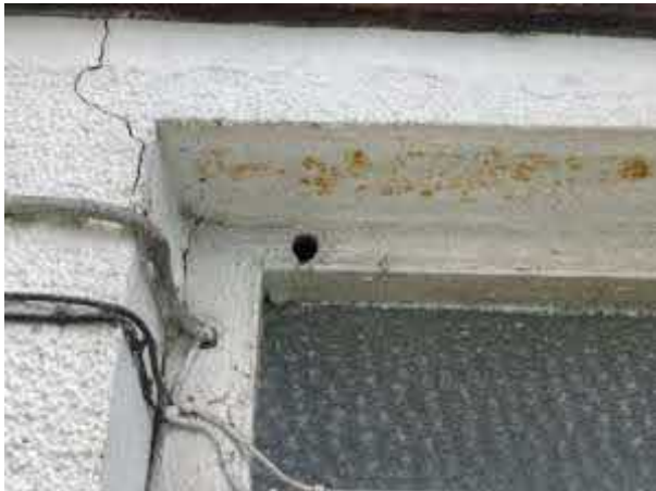
Photo 17: Hole within Wooden Window Frame – B1
