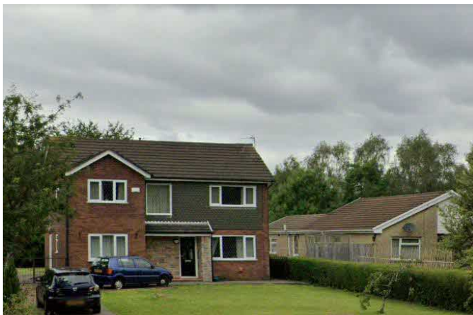
Photo 6: Houses in Victoria Street near to site
