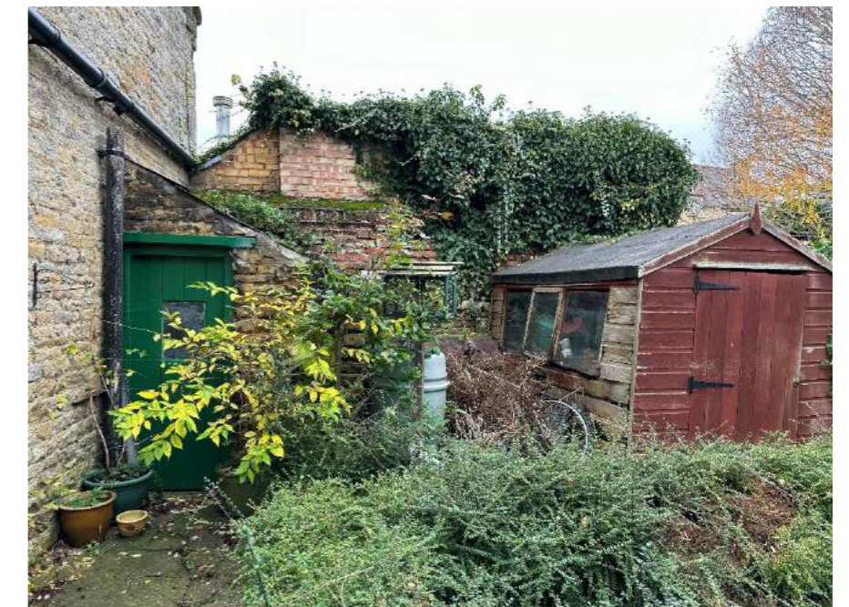
Fig 3. Courtyard/garden area - existing garden stores and outdoor WC
