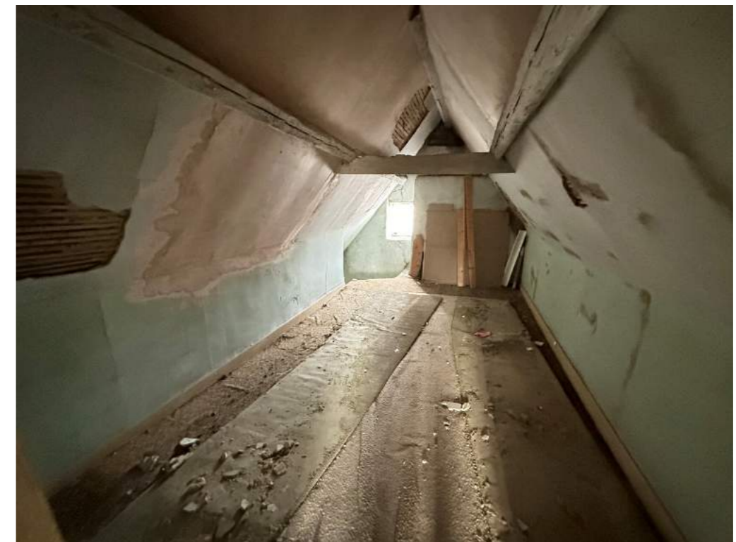
Fig 10. Second floor level
