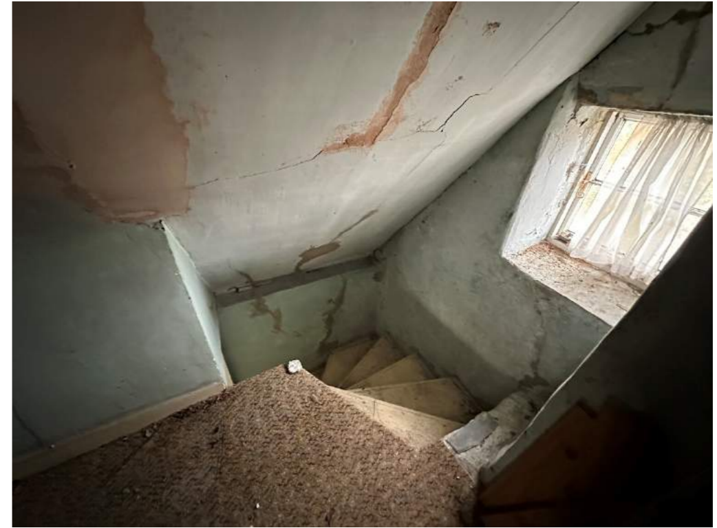
Fig 9. Staircase to second floor level
