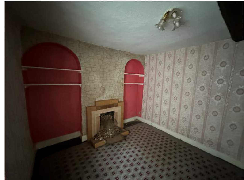
Fig 7. Existing ground floor South side reception room
