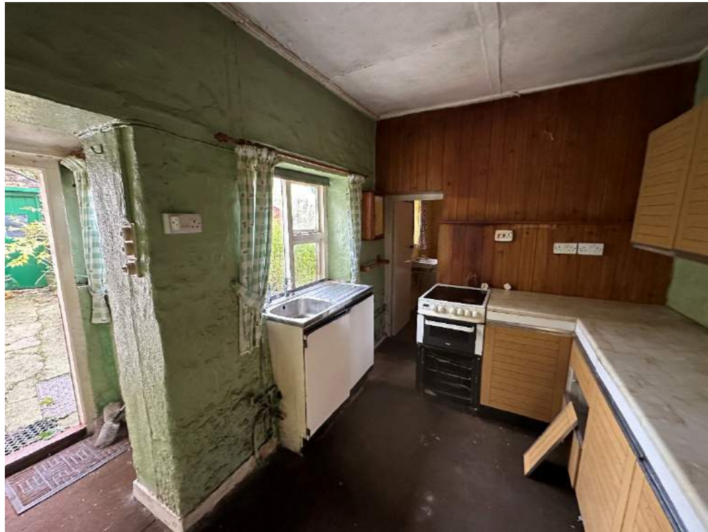
Fig 4. Existing kitchen and porch area leading to garden.
