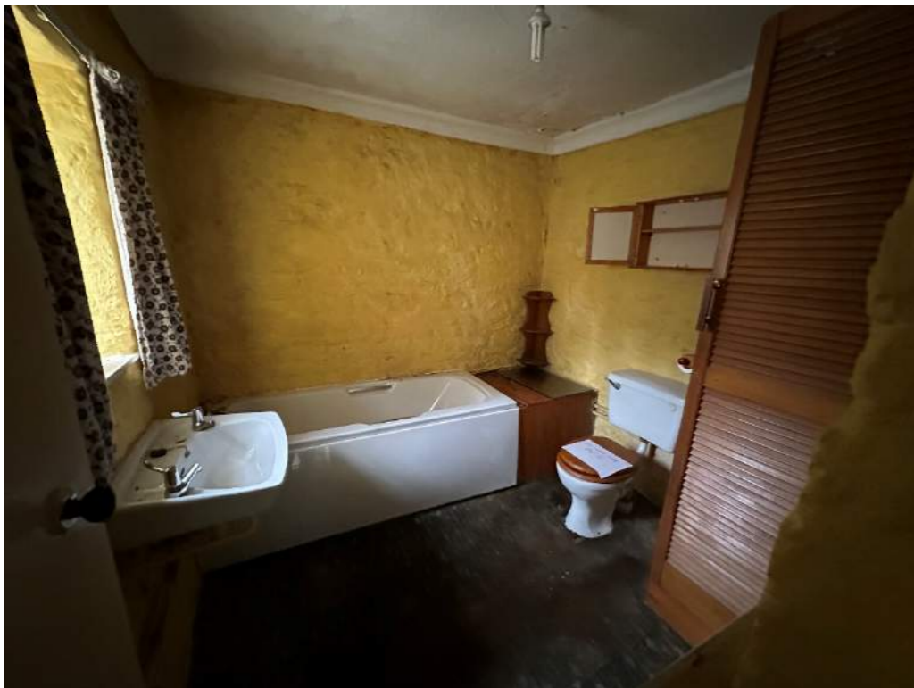
Fig 5. Existing ground floor bathroom
