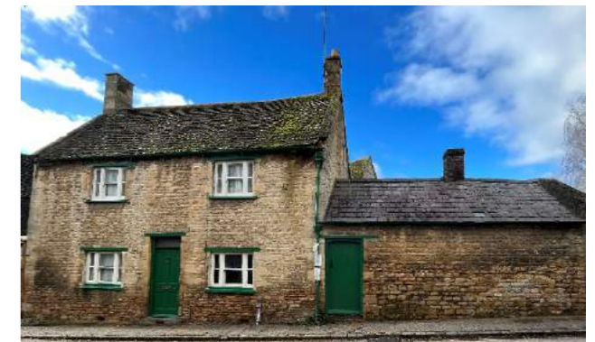
Fig 28. Existing green joinery
