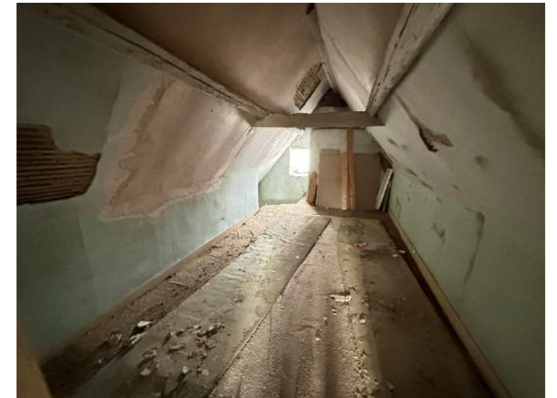
Fig 25. Existing attic room - to be bedroom
