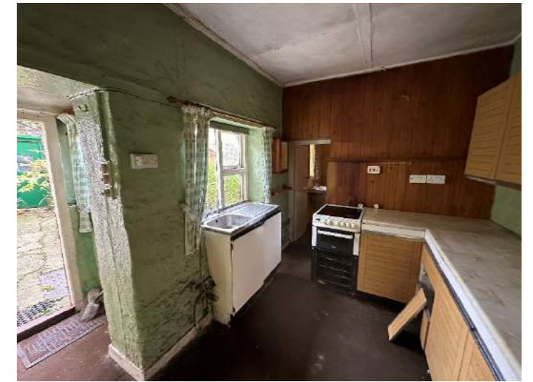
Fig 20. Chimney breast to be removed
