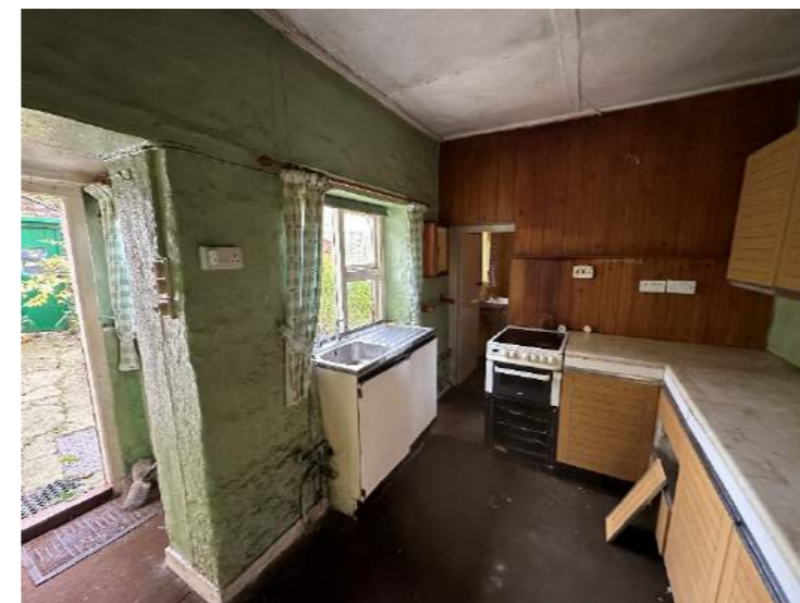
Fig 10. Ground Floor Kitchen leading to bathroom.
