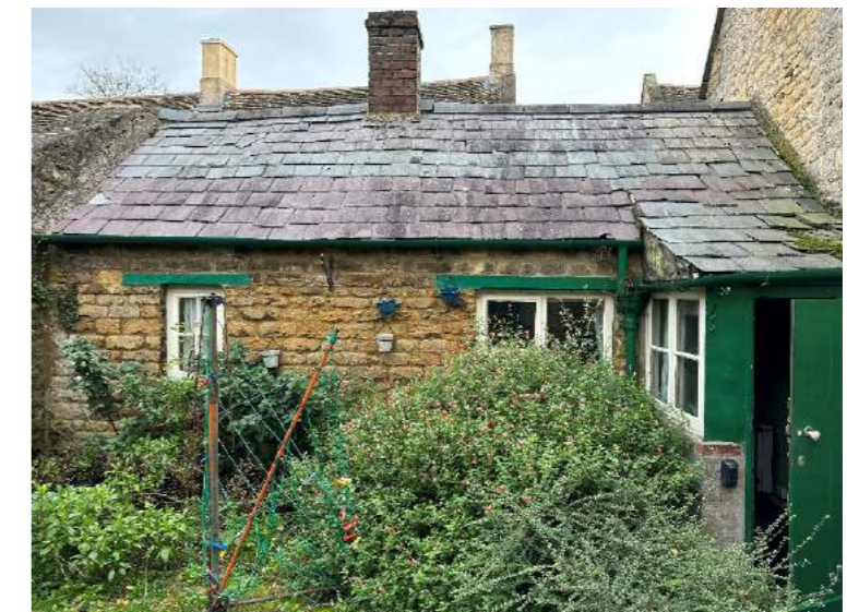
Fig 31. Existing courtyard area
