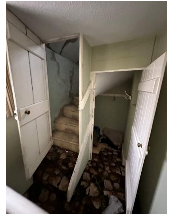
Fig 23. Existing door to attic stair
