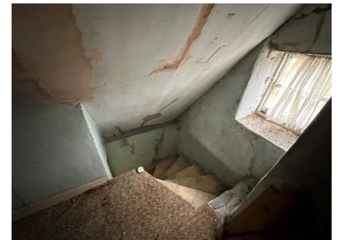
Fig 24. Existing attic stair/landing
