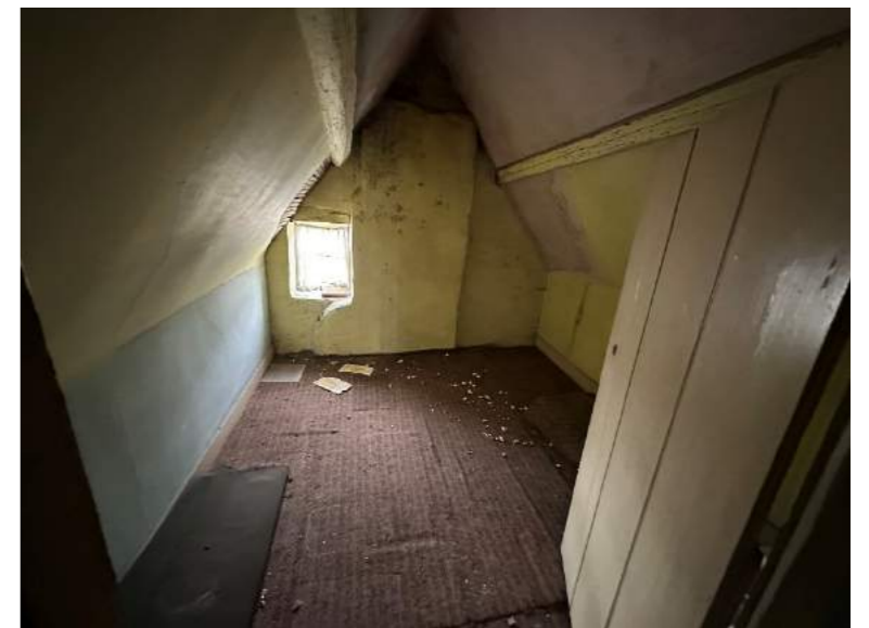
Fig 26. Existing attic room - to be converted into ensuite
