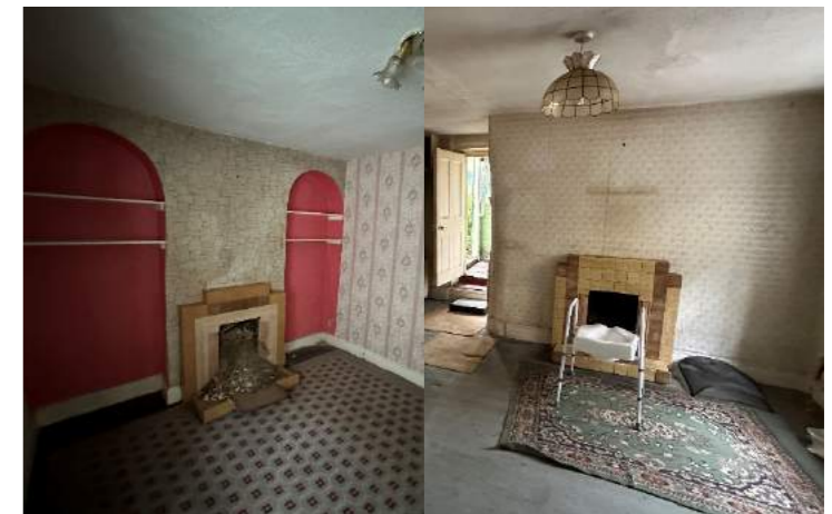
Fig 21. Fire surrounds In Ground Floor reception rooms
