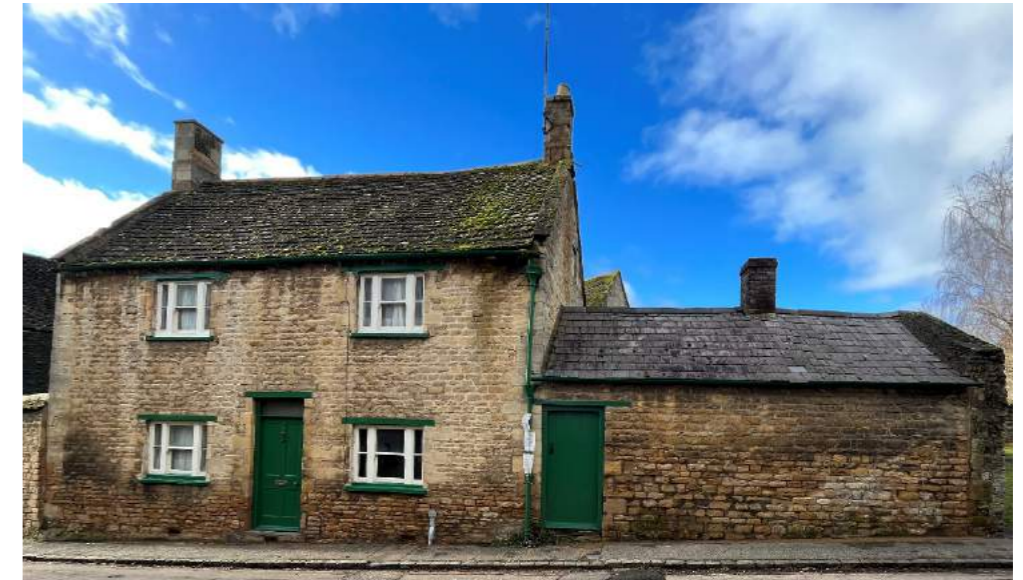
Fig 6. White Cottage Elevation from Park Street
