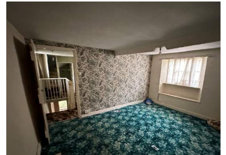
Fig 22. Door leading to First Floor bedroom to be removed
