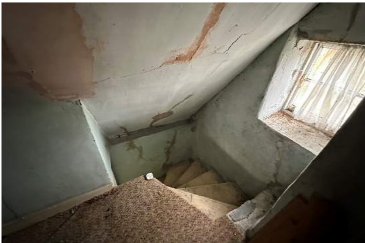
Fig 13. Second floor stair
