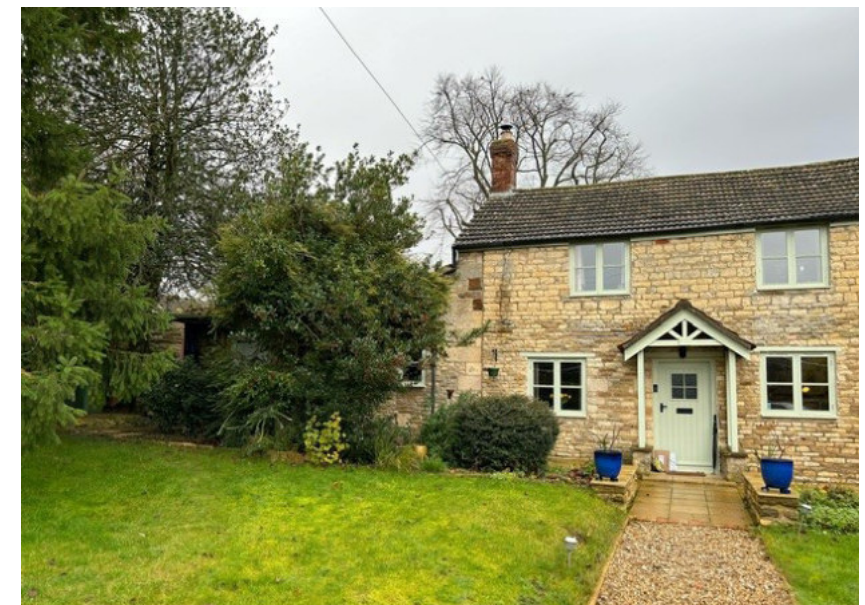
Fig 12A. Image of the Anchorage's front(north) elevation showing T1 and T2 9
