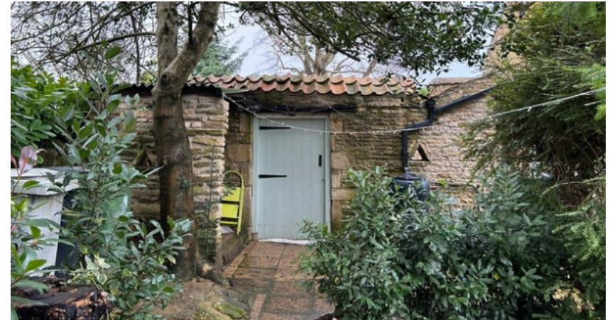
Fig 06A. View of Existing Courtyard Door from North Looking South
