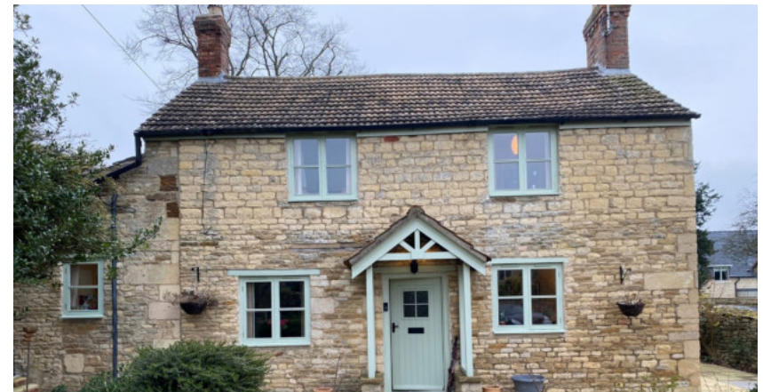
Fig 06B. View of Existing Front (North) Elevation from Driveway
