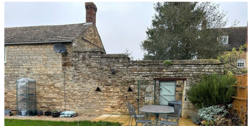
Fig 06C. View of Existing Courtyard Door from North Looking South
