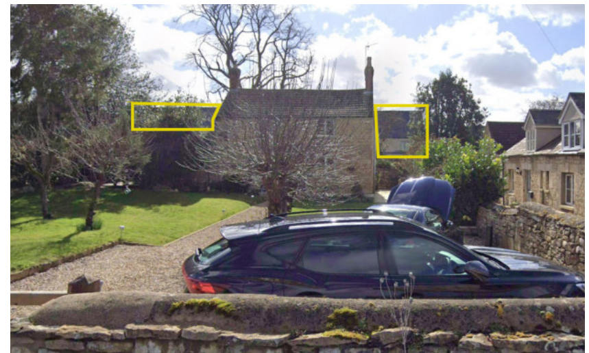
Fig 14E. Street View Facing South of The Site - Highlighted Glebe Road Development
