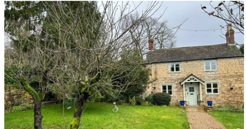
Fig. 5A. Existing Image of Front (north) Elevation
