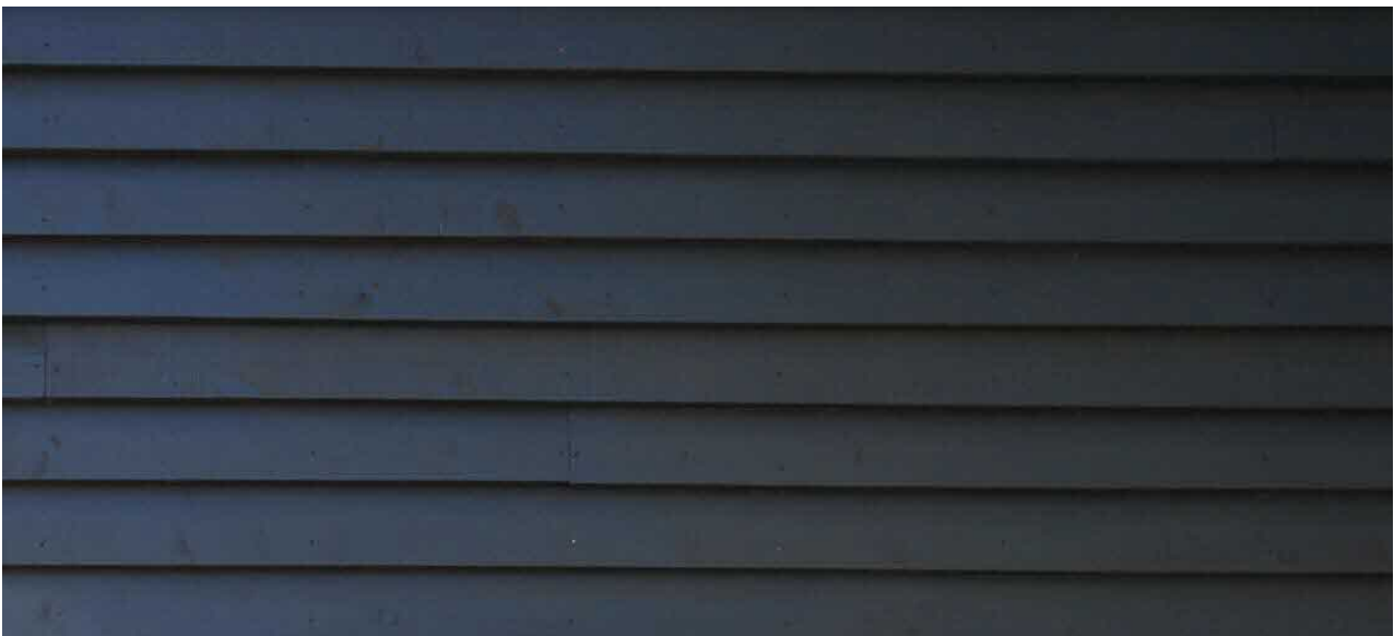
Sample image showing horizontal profile weatherboard
