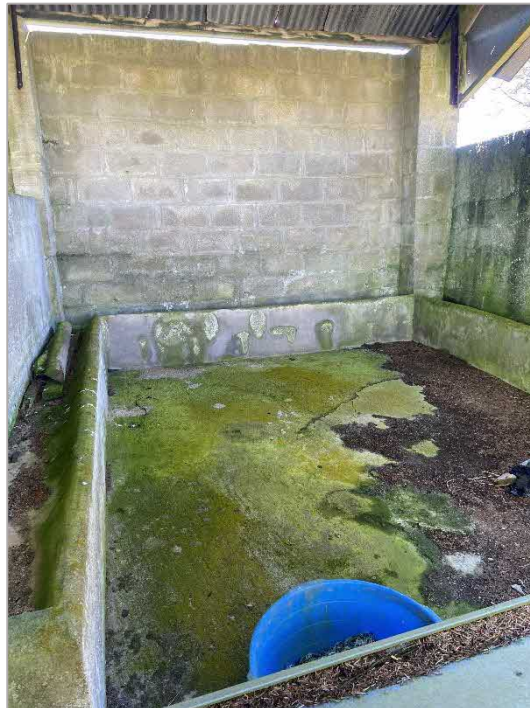
PHOTOGRAPH 8: View of the western interior of the building on site
