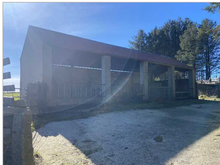
PHOTOGRAPH 4: View of the northern side of the building on site with its concrete yard in the foreground
