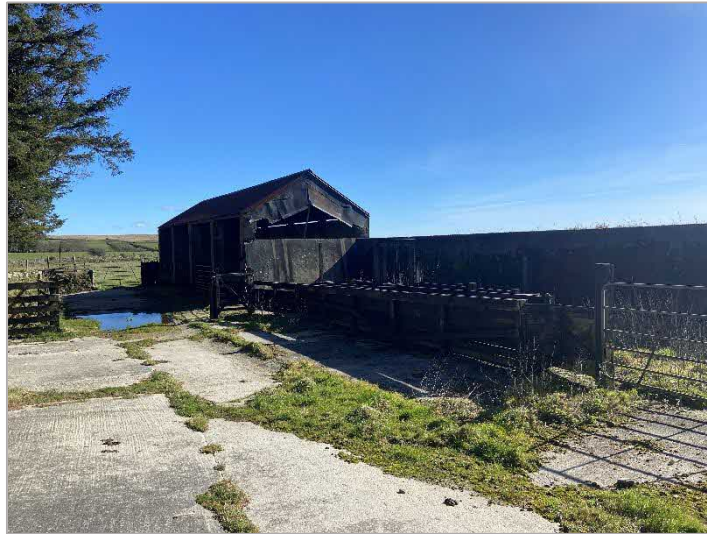
PHOTOGRAPH 5: View across the site's yard towards the east
