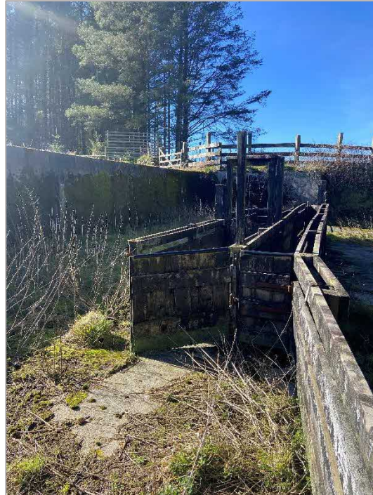
PHOTOGRAPH 6: View of an animal pen on site
