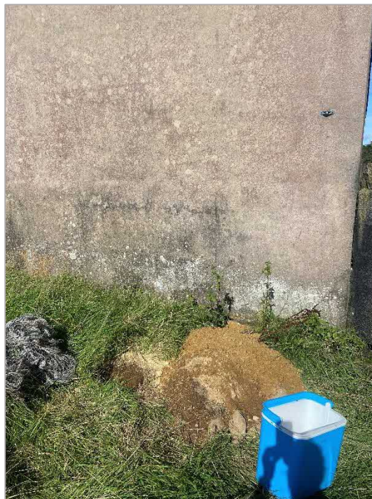
PHOTOGRAPH 4: View of the trial pit's location
