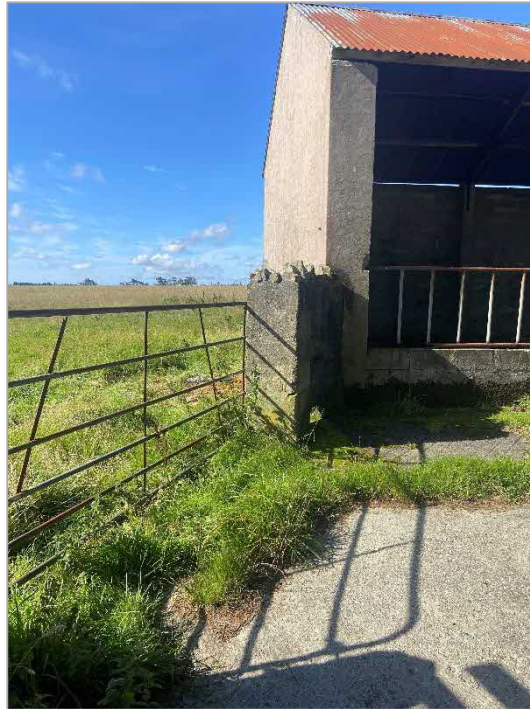
PHOTOGRAPH 1: View of the trial pit's location immediately adjacent to the south-eastern gable end of the building
