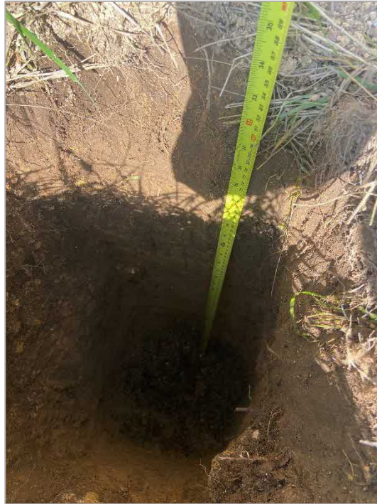
PHOTOGRAPH 3: View of the trial pit
