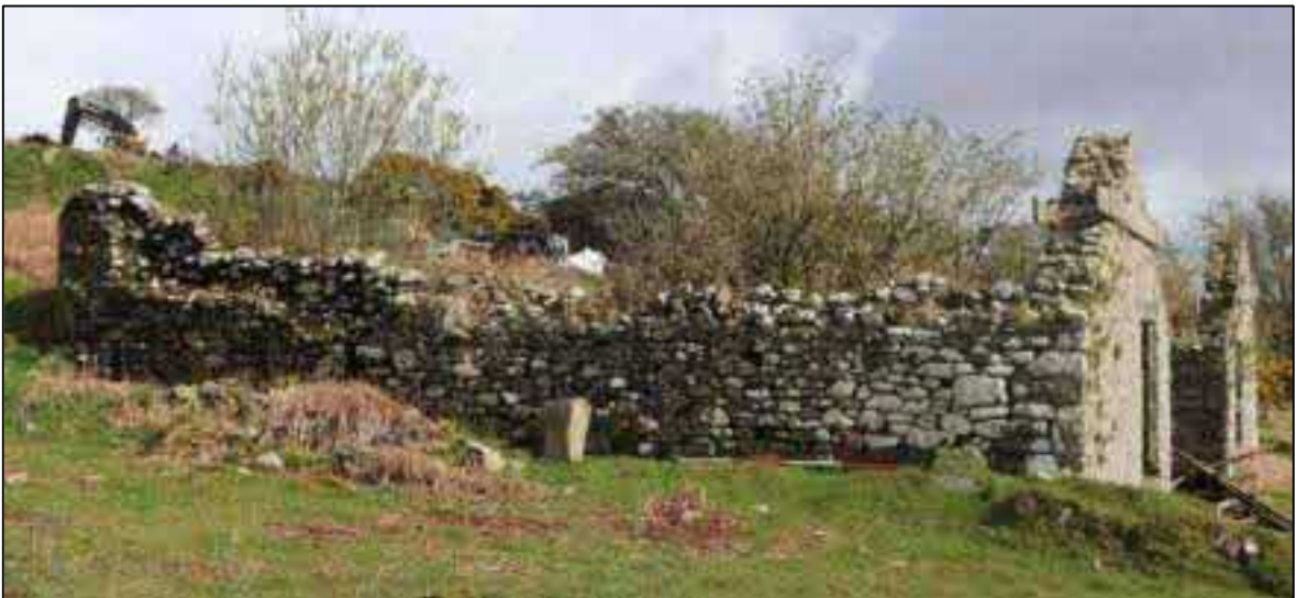
FIGURE 21: THE SOUTH-WEST ELEVATION; VIEWED FROM THE SOUTH (SCALE 2M).
