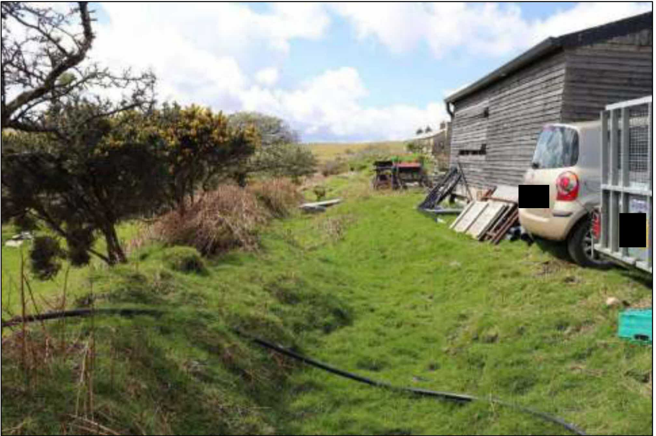
63. THE HEDGE BANK LOOKING TOWARDS BARN; VIEWED FROM THE NORTH.
