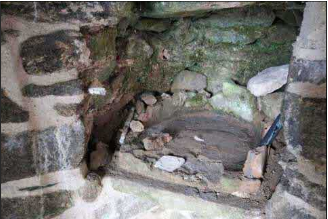
56. THE DETAIL OF DAMAGED CLOAM OVEN.
