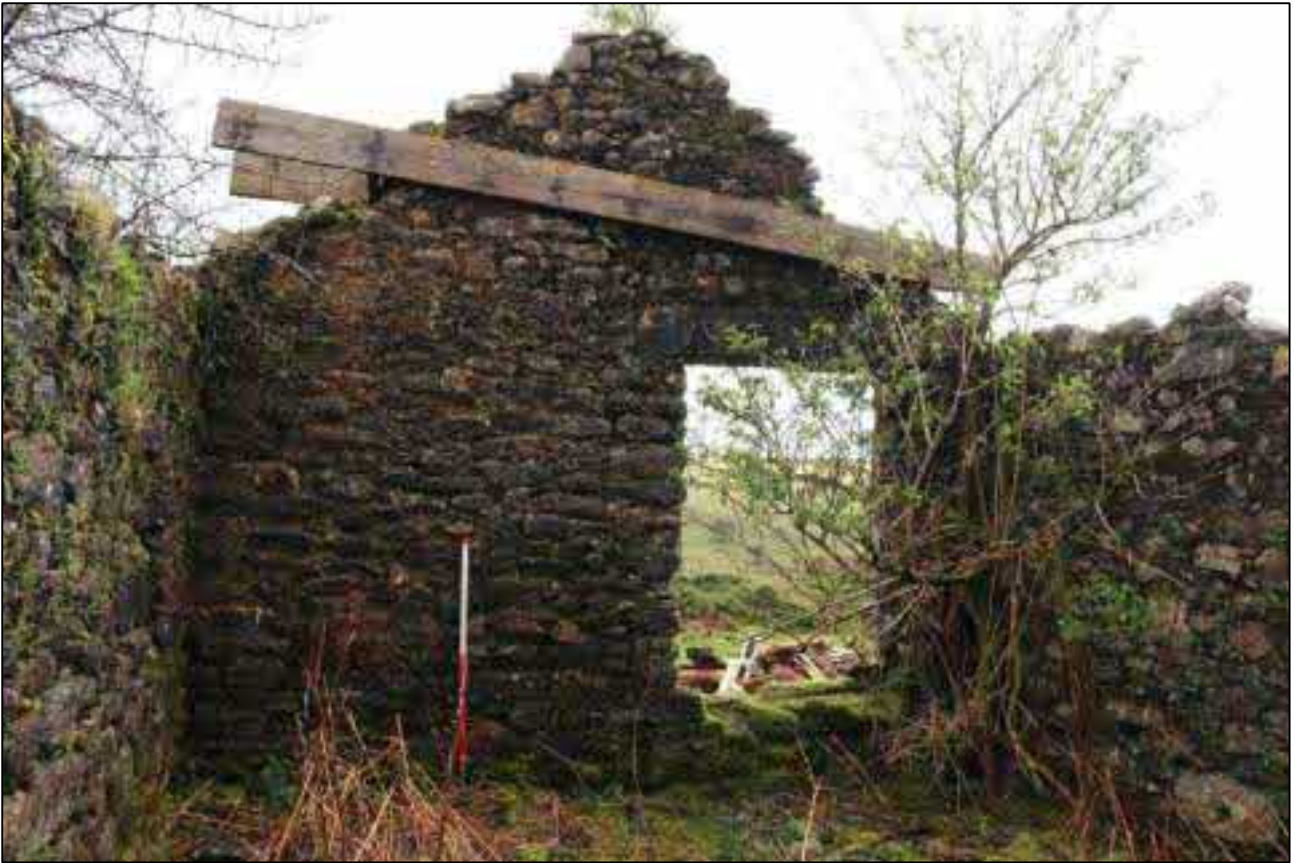
25. THE EAST INTERNAL ELEVATION OF B1C; VIEWED FROM THE WEST (SCALE 1M).
