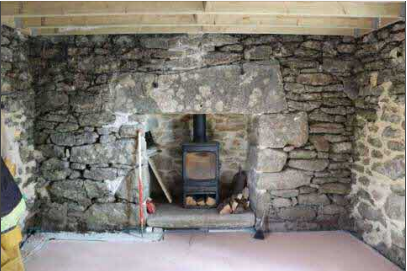
49. THE FIREPLACE IN THE NORTHERN ROOM OF THE HOUSE, CLOAM OVEN TO LEFT SIDE; VIEWED FROM THE SOUTH (SCALE 1M).
