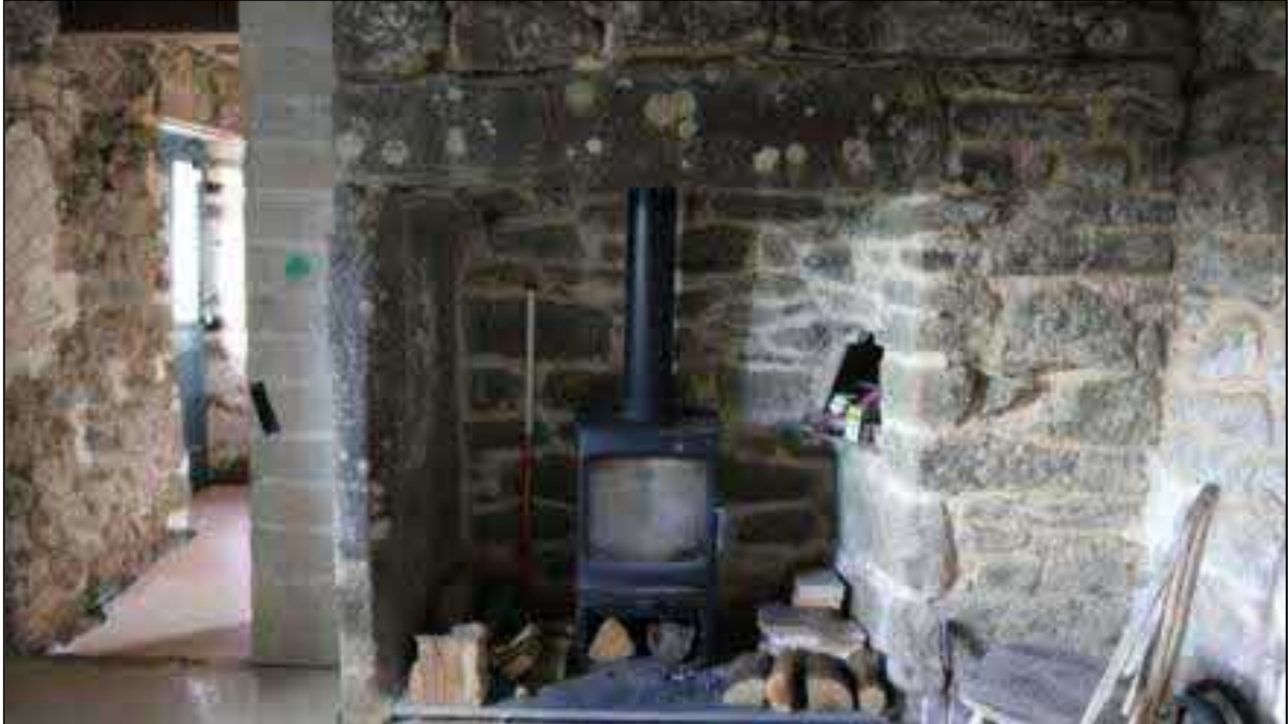
FIGURE 27: CHAMFERED FIRE SURROUND SEEN TO CENTRAL BAY OF HOUSE; VIEWED FROM THE NORTH (SCALE 1M).
