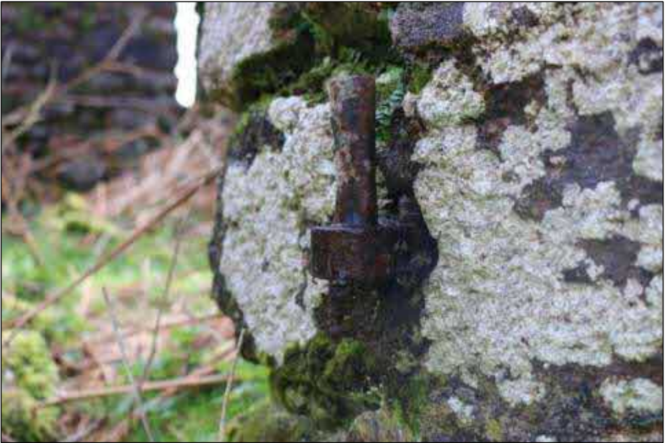
7. HEAVY PINTLE SURVIVING TO NORTH SIDE OF D3.
