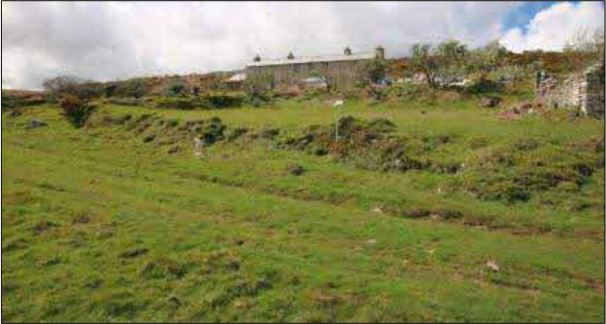
FIGURE 14: VIEW ACROSS THE FORMER GARDEN ATTACHED TO THE HOUSE (BARN TO THE RIGHT); VIEWED FROM THE SOUTH-EAST (SCALE 1M)
