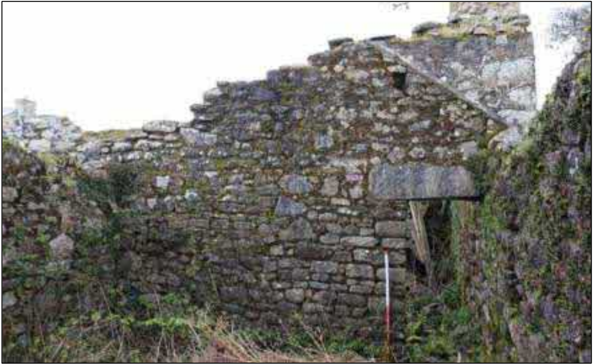
FIGURE 26: THE INTERIOR OF B1C; VIEWED FROM THE EAST (SCALE 1M).
