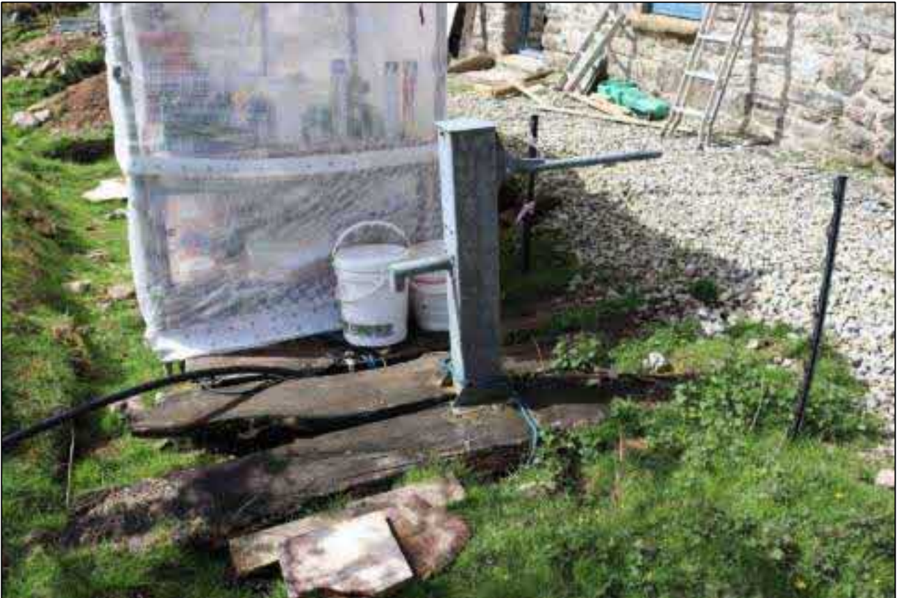
57. A DEEP WELL COVERED, LOCATED TO THE NORTH OF THE HOUSE AGAINST EAST ELEVATION; VIEWED FROM THE NORTH.
