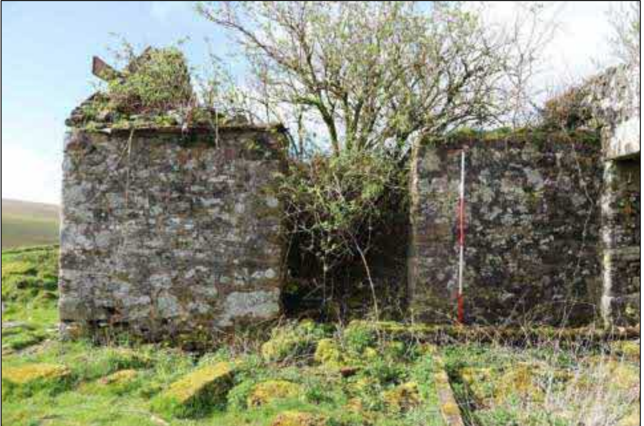
8. D4 LEADING TO B1B; VIEWED FROM THE NORTH (SCALE 2M).
