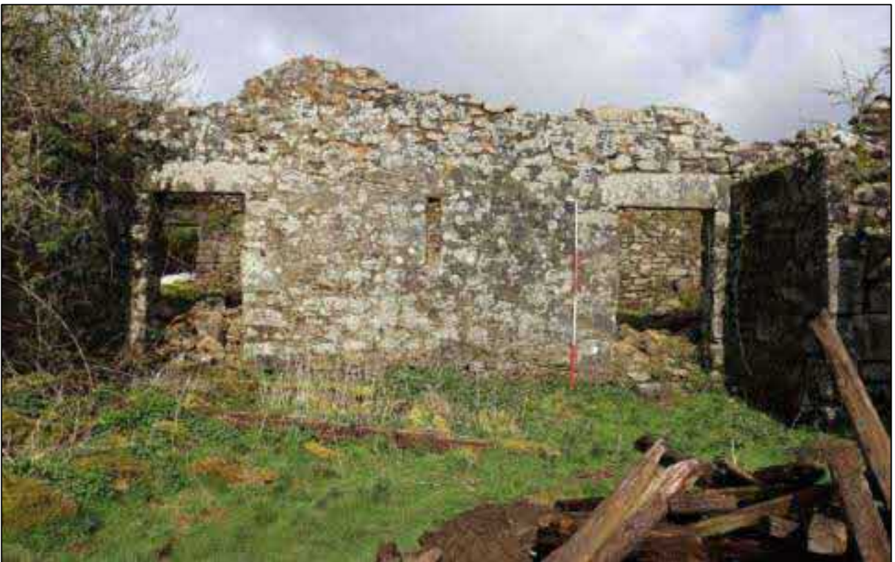
4. THE EAST FRONT OF B1A WITH SYMMETRICALLY PLACED DOORS WITH SLIT VENT BETWEEN; VIEWED FROM THE EAST (SCALE 2M).
