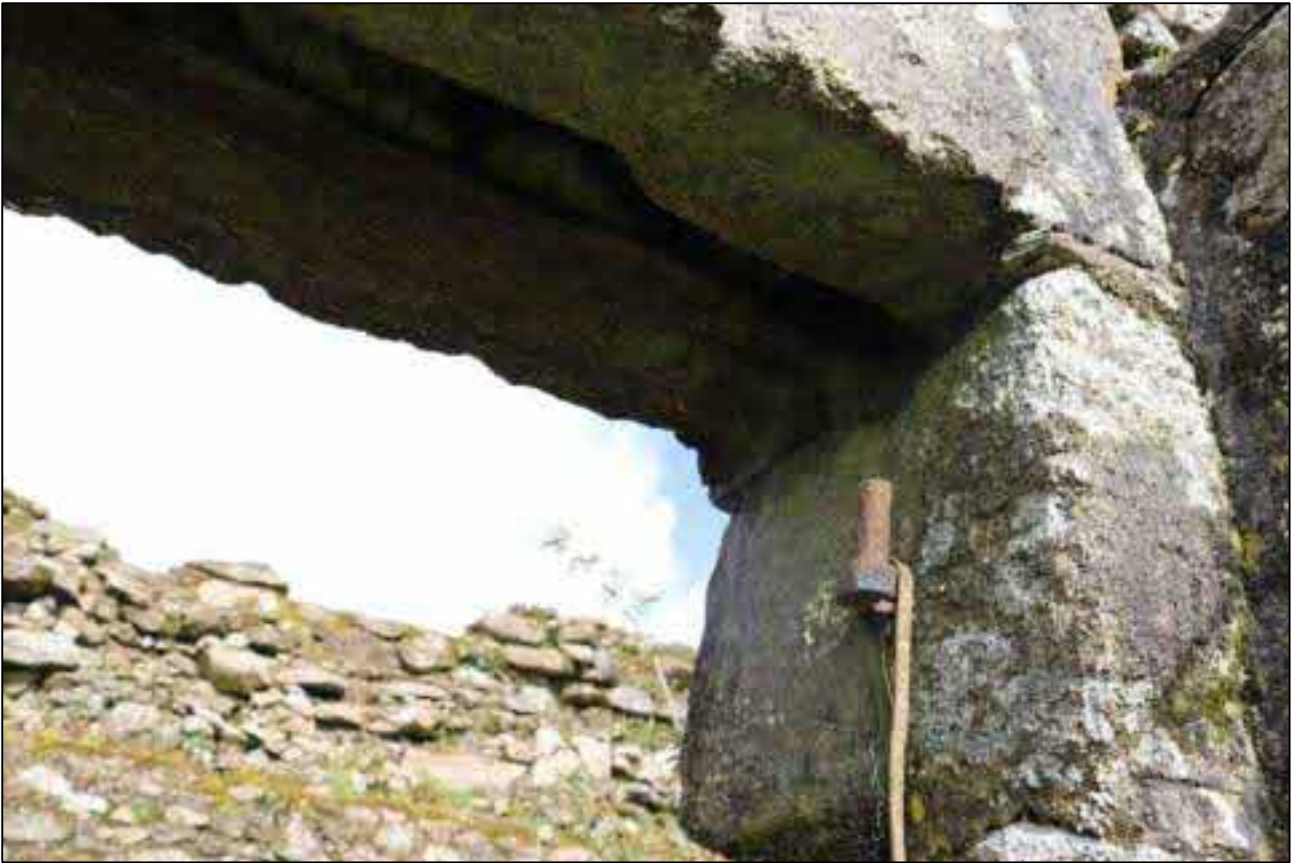
5. LINTEL AND IRON BRACE SEEN TO D2 WITH HEAVY PINTLE SURVIVING TO NORTH SIDE.
