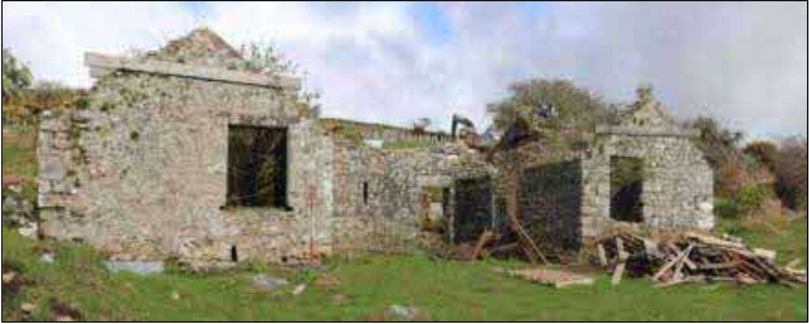
FIGURE 22: THE SOUTH-EAST ELEVATION; VIEWED FROM THE SOUTH-EAST (SCALE 2M).
