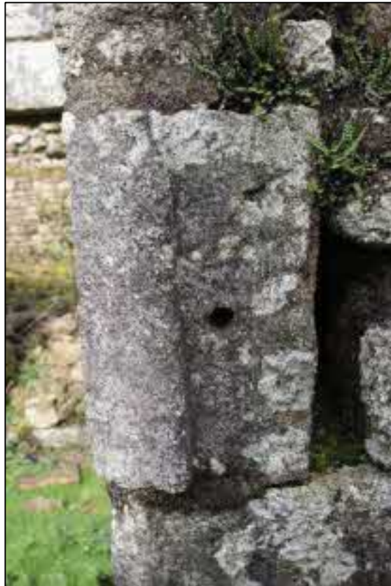
5. LINTEL AND IRON BRACE SEEN TO D2 WITH HEAVY PINTLE SURVIVING TO NORTH SIDE.
