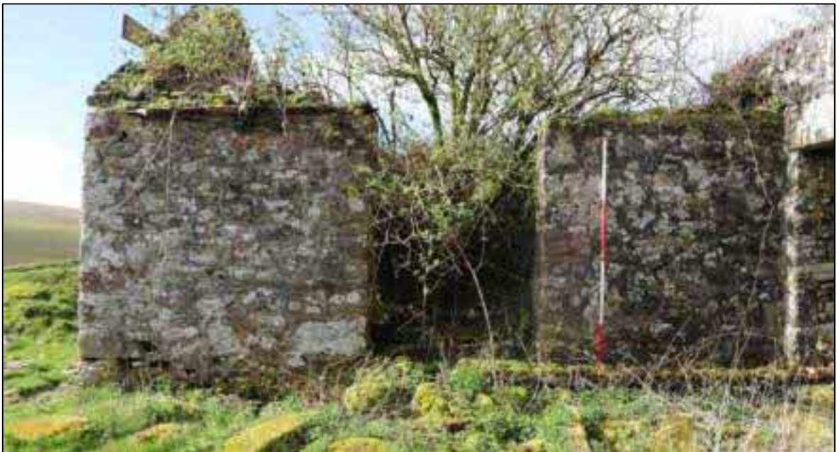
FIGURE 25: D4 INTO B1B; VIEWED NORTH-EAST (SCALE 2M).
