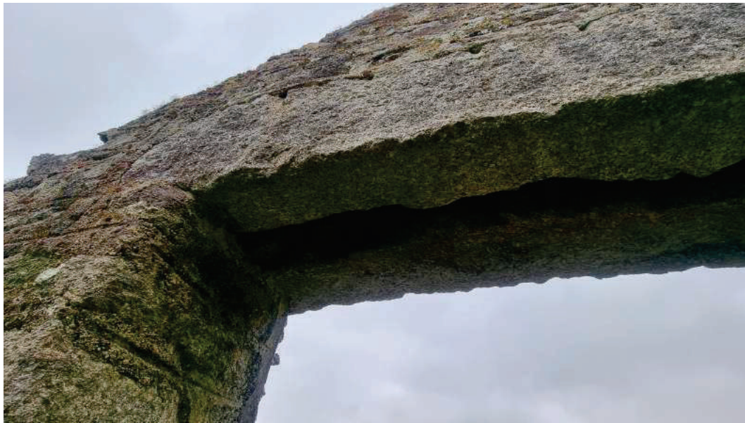
Photograph 14.0 – Granite lintels visible from underside [gable opening]
