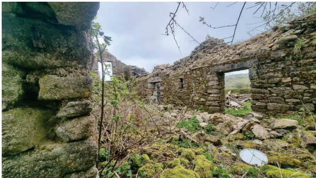
Photograph 11.0 - Internal floor concealed from rubble and foliage build up
