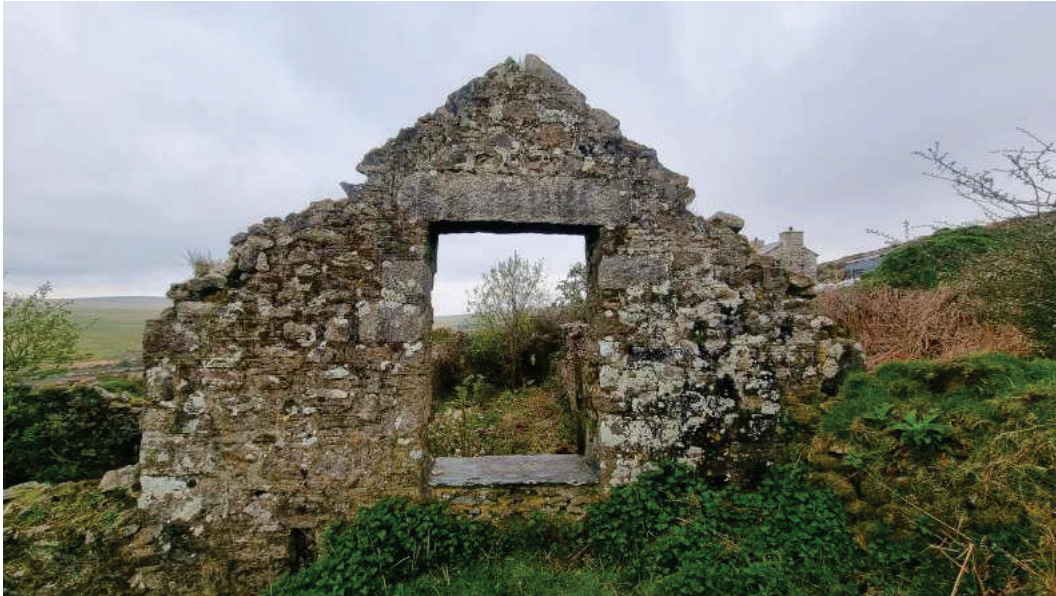
Photograph 12.0 – Possible first floor opening to northern gable wall
