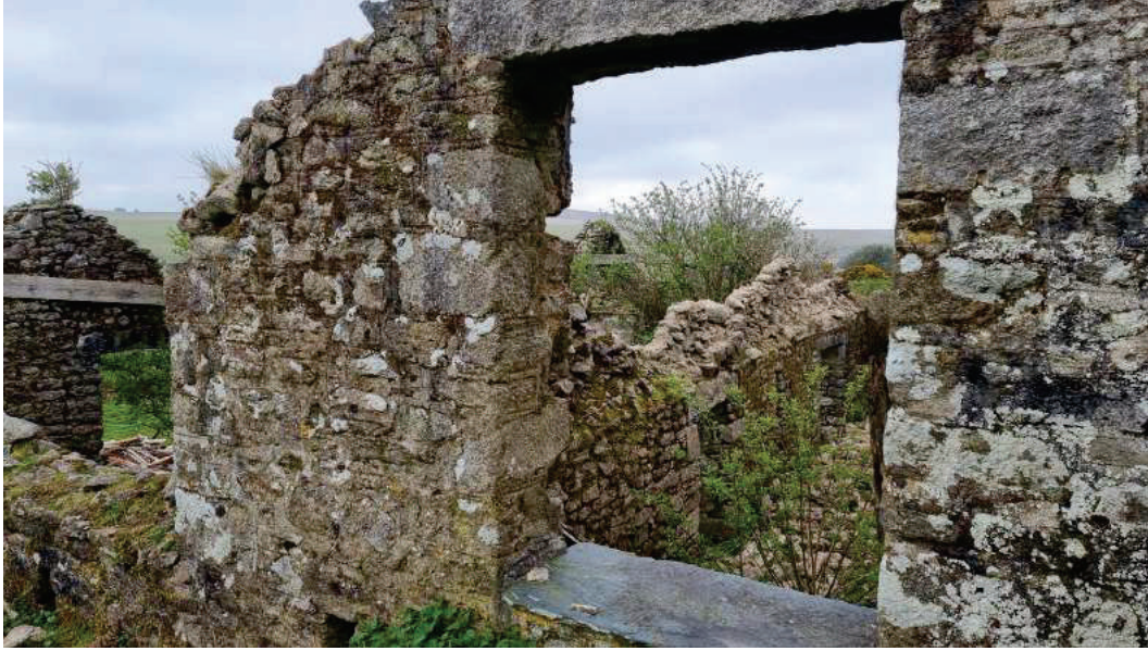
Photograph 2.0 – Granite quins, jambs and lintels
