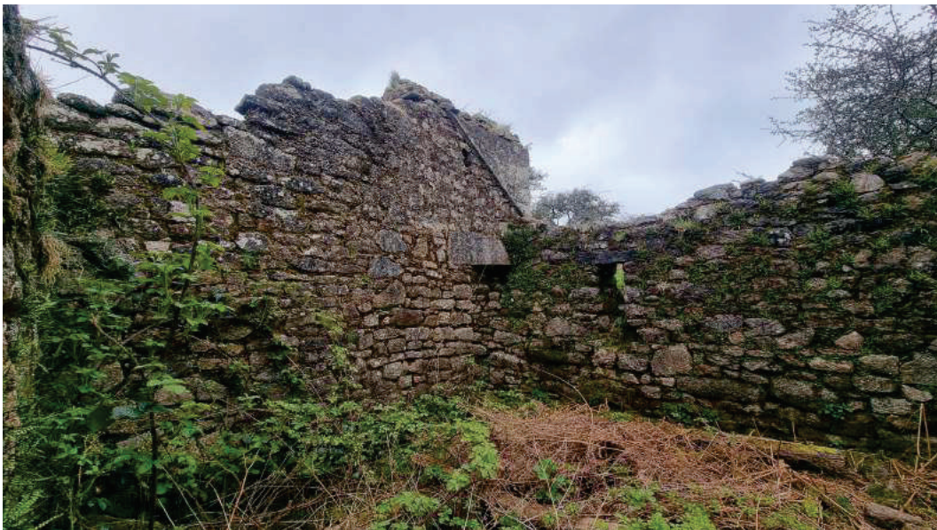
Photograph 4.0 – Exposed head of masonry throughout building
