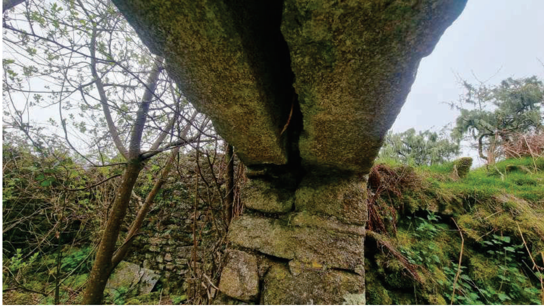
Photograph 13.0 – Granite lintels visible from underside [ground floor opening]
