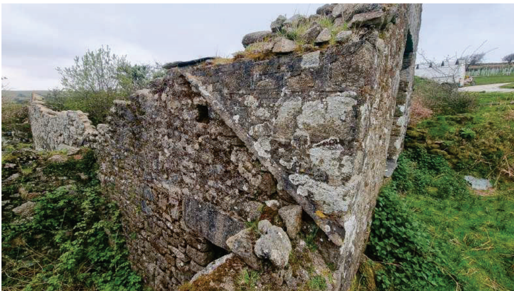
Photograph 6.0 - Cementitious mortar and flashing
