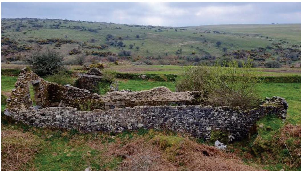
Photograph 1.0 – Lack of roof structure to building
