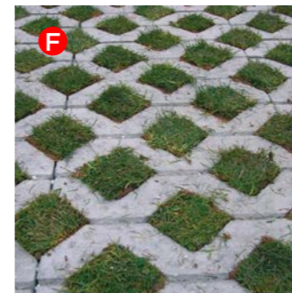
F GrassPark Permeable Paving Grid - Part of Sustainable Urban Drainage (SUDS)
