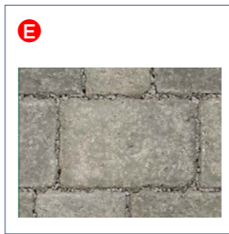
E Permeable Block Paver Part of Sustainable Urban Drainage (SUDS)
