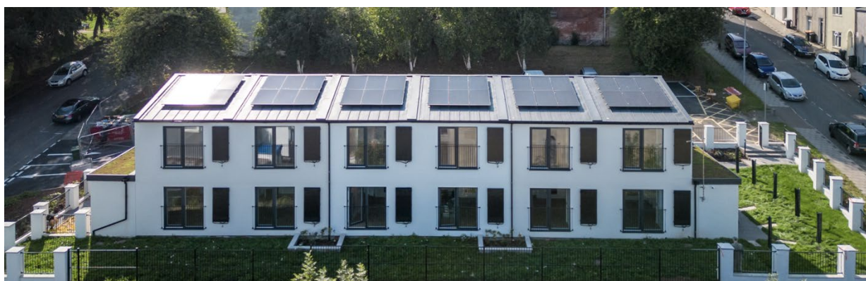
Roof Mounted Photovoltaic Panels and Solar Assisted heat pump panels at the ZED PODs scheme in Newport, Wales
