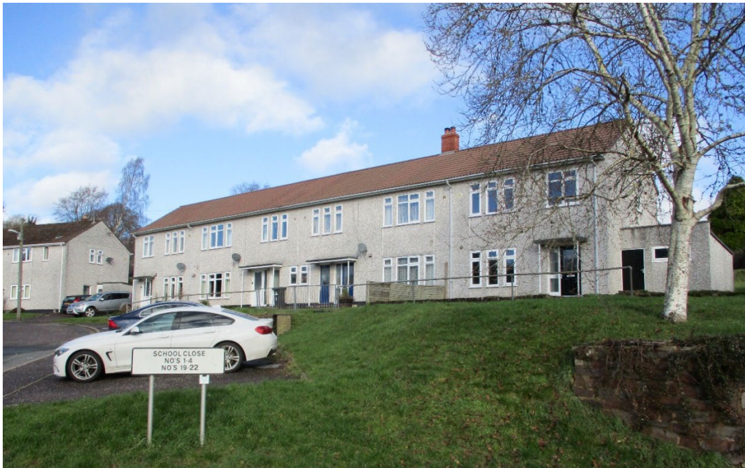
Photo 1: View of the Site.
