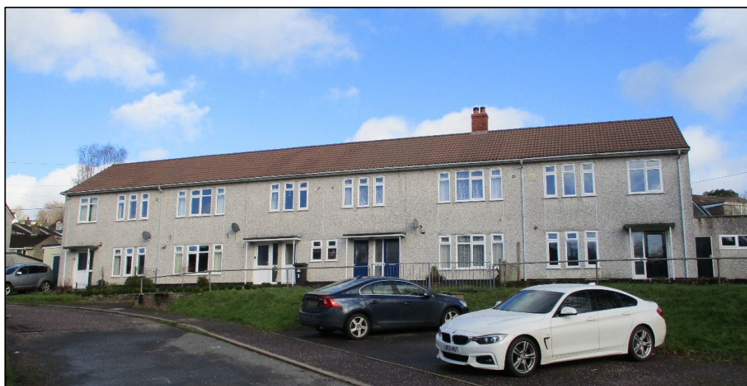
Photo 8: 4 (l.) to 7 (r.) School Close. Looking north-east from School Close.
