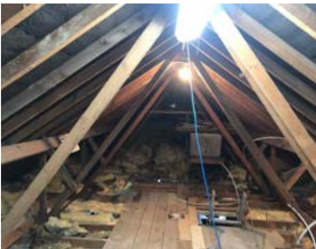
Image 5: View of the loft void at the western gable.
