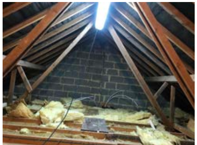
Image 6: View of the void facing the eastern gable.
