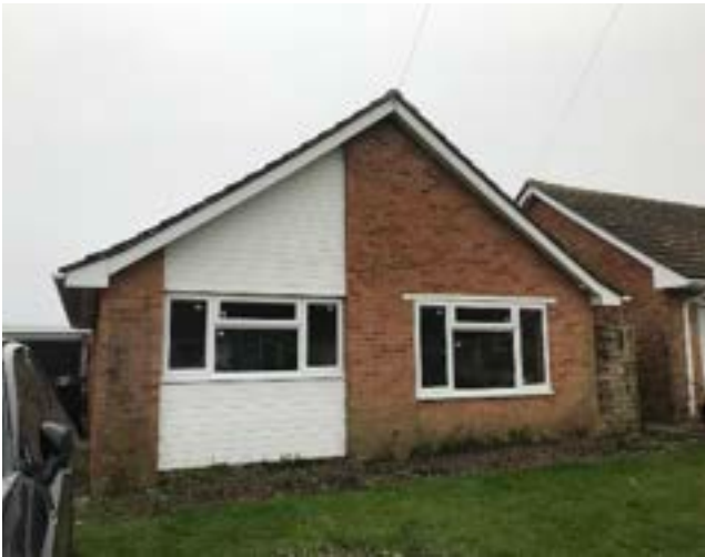
Image 1: View of the eastern gable end of the building.
