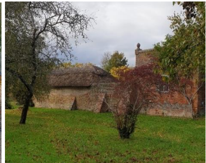
Rear view of existing outbuilding
