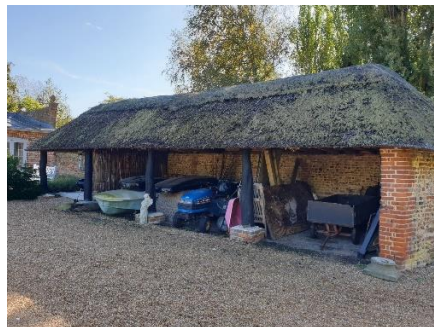
Front view of existing outbuilding
