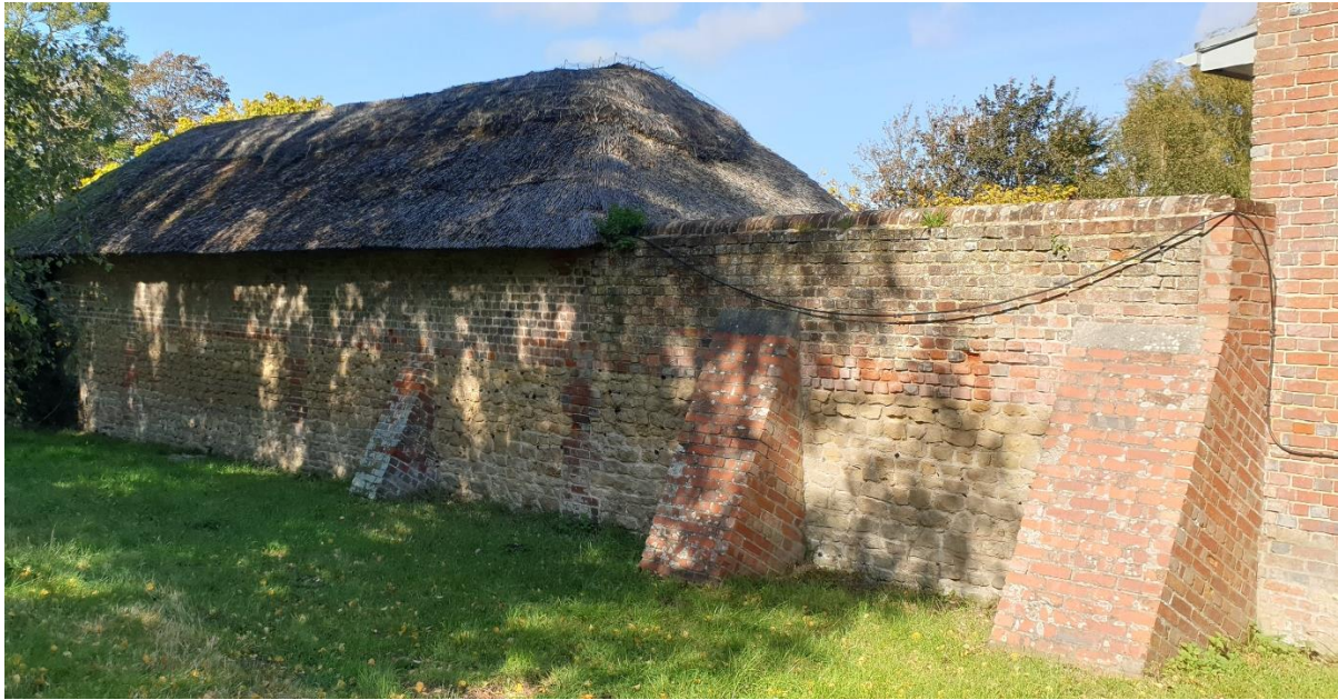
Southern view of outbuilding and its three existing buttresses
