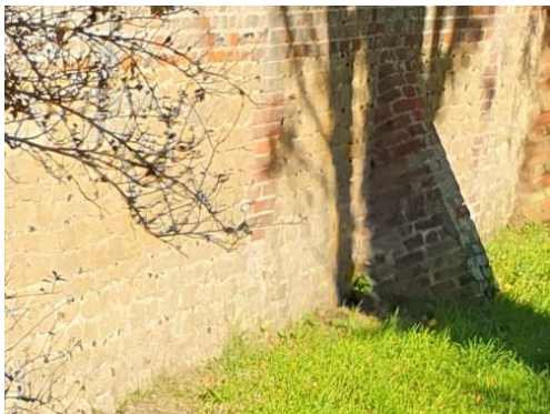
Rear view of outbuilding - existing partial stone with later additions of brick.
