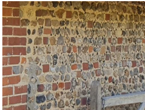
Side view of outbuilding- flint and brick wall
