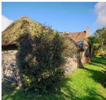
Rear view of existing outbuilding
