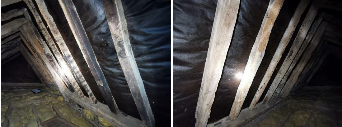
Figure 68. View of the roofing felt
