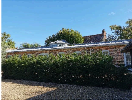
Figure 80. View of the western elevation of the annex
