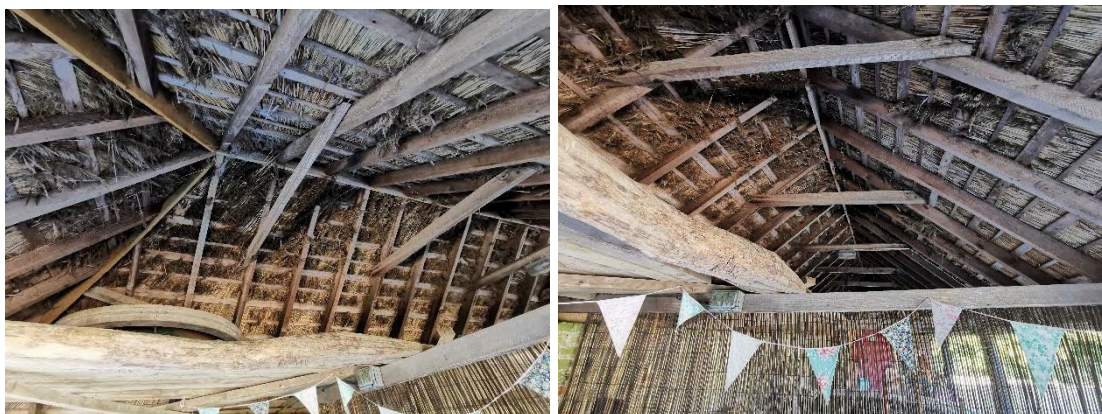
Figure 85. View of the roof of the thatched carport
