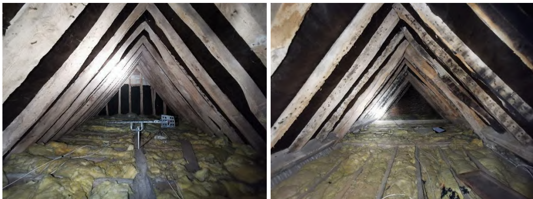
Figure 66. Internal view of the loft void
