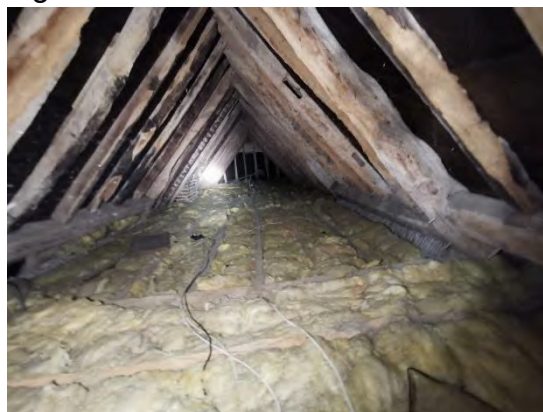
Figure 67. Internal view of the loft void
