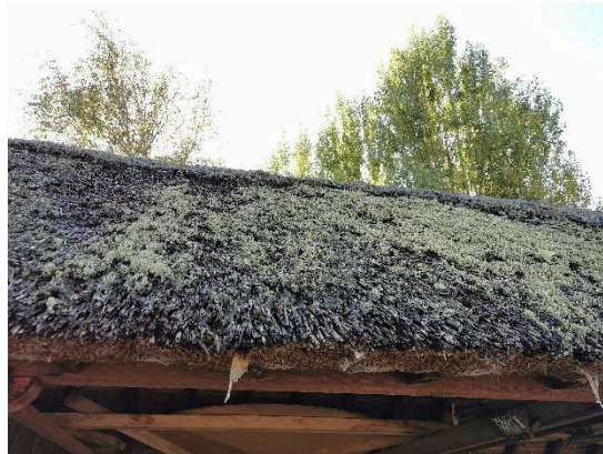
Figure 84. View of the of the thatched roof of the carport
