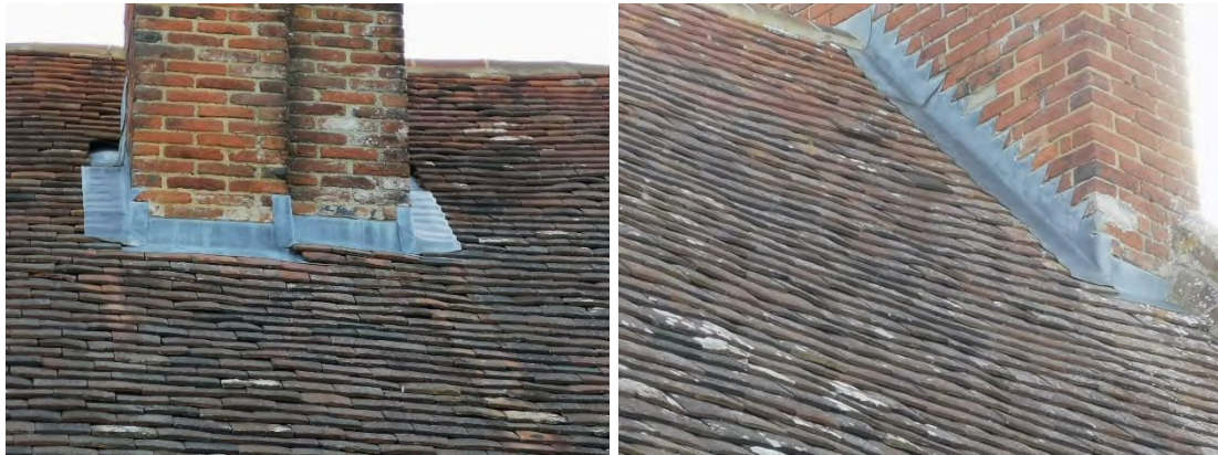
Figure 62. View of the lead flashing around the base of the chimney
