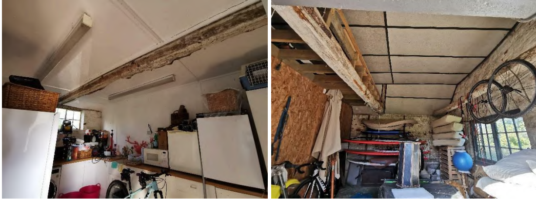
Figure 77. Internal view of the garage
