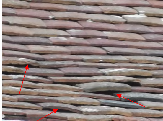
Figure 58. Example of lifted roof tiles
