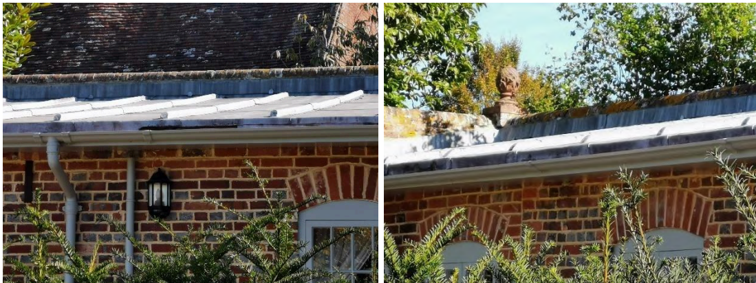
Figure 81. View of the lead roof
