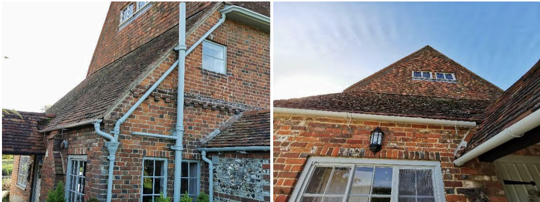
Figure 55. View of the northern lean-to extension
