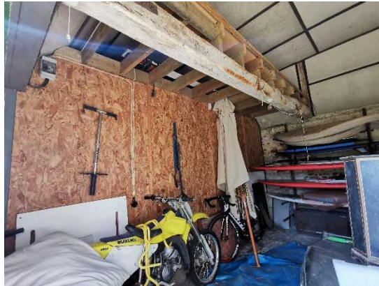
Figure 78. Internal view of the garage
