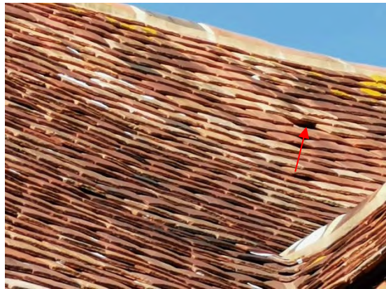
Figure 60. Example of lifted roof tiles
