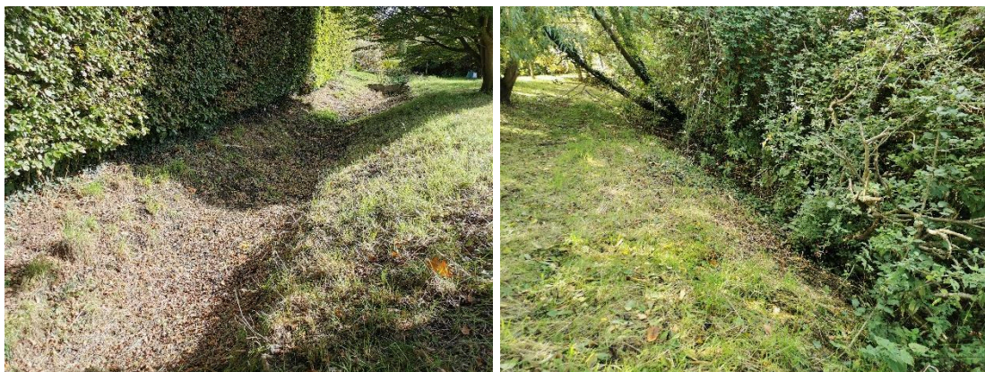
Figure 26. View of the dry ditch on site
