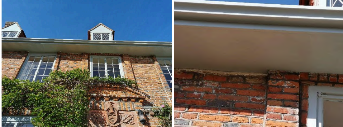
Figure 65. View of the tightly fitted soffit
