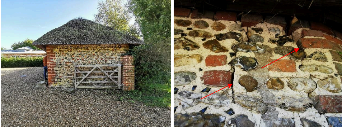
Figure 86. View of the western wall of the thatched carport
