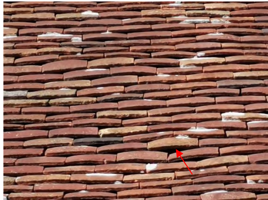
Figure 59. Example of lifted roof tiles
