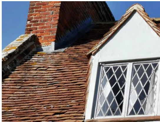
Figure 63. View of the lead flashing around the base of the chimney
