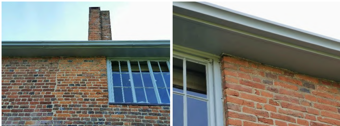
Figure 64. View of the tightly fitted soffit
