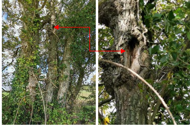
Figure 92. Another oak tree along the western boundary of the southern grass field with a wound – moderate bat potential
