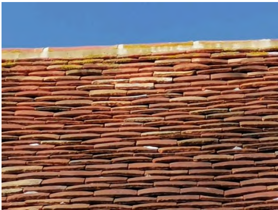
Figure 60. Example of lifted roof tiles
