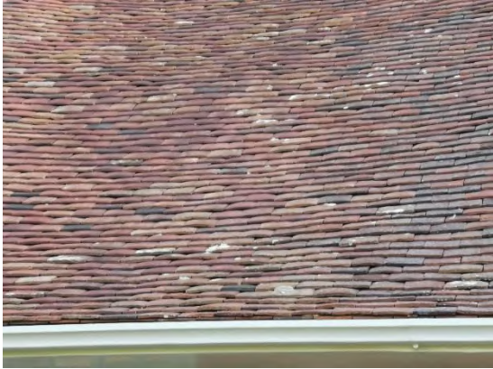
Figure 58. Example of lifted roof tiles
