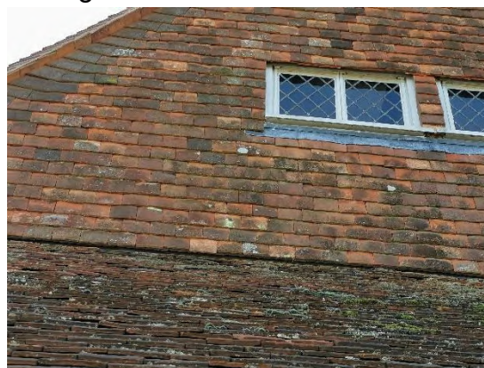
Figure 57. View of the northern gable-end hanging tiles
