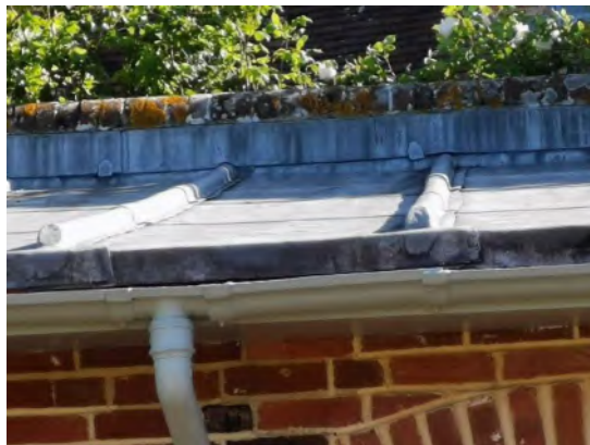
Figure 82. View of the lead roof
