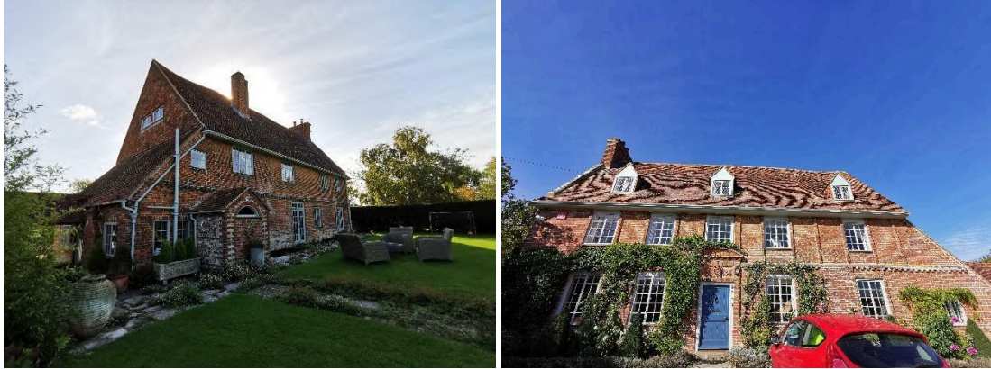
Figure 54. View of the eastern (right) and western (left) elevations of the Old Manor House
