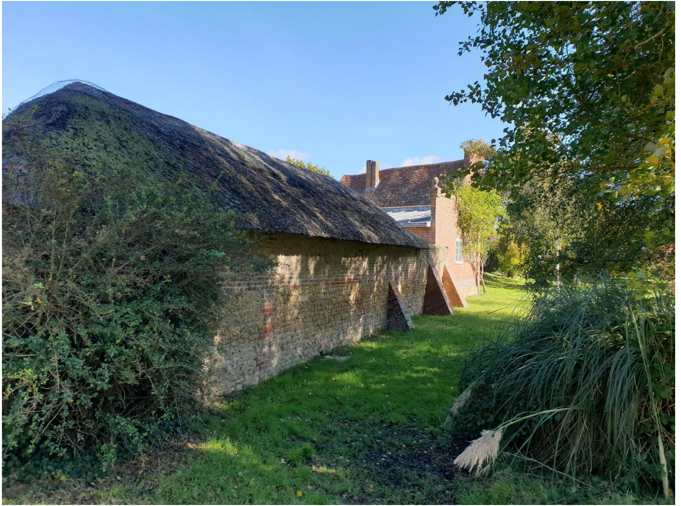
Fig 10 Cart barn historic wall (west)
