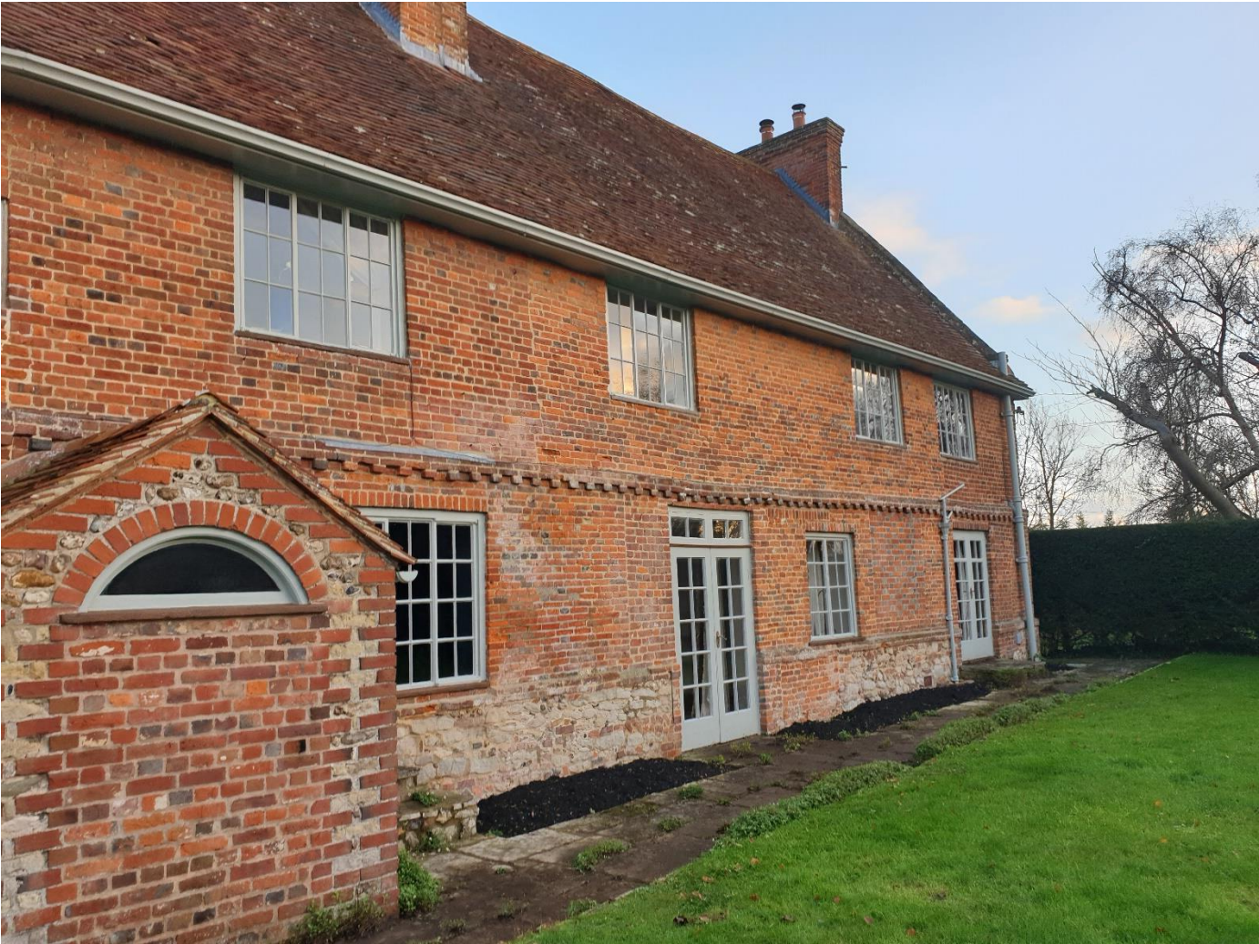
Fig 6 North elevation with bricked in porch
