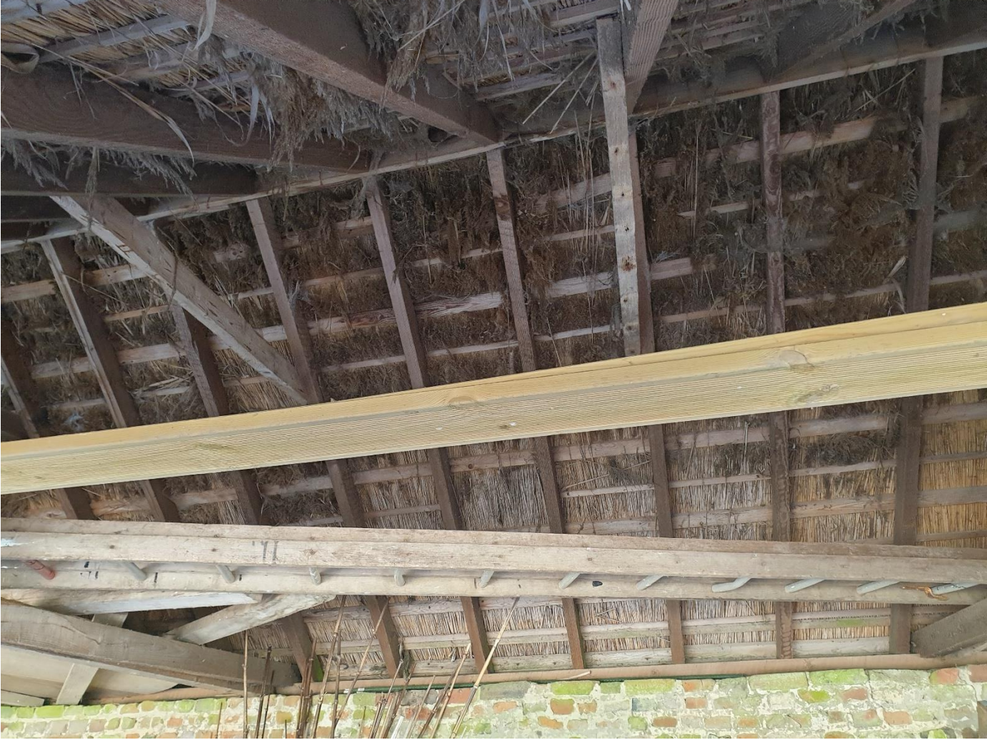
Fig9 Cart barn modern roof timbers
