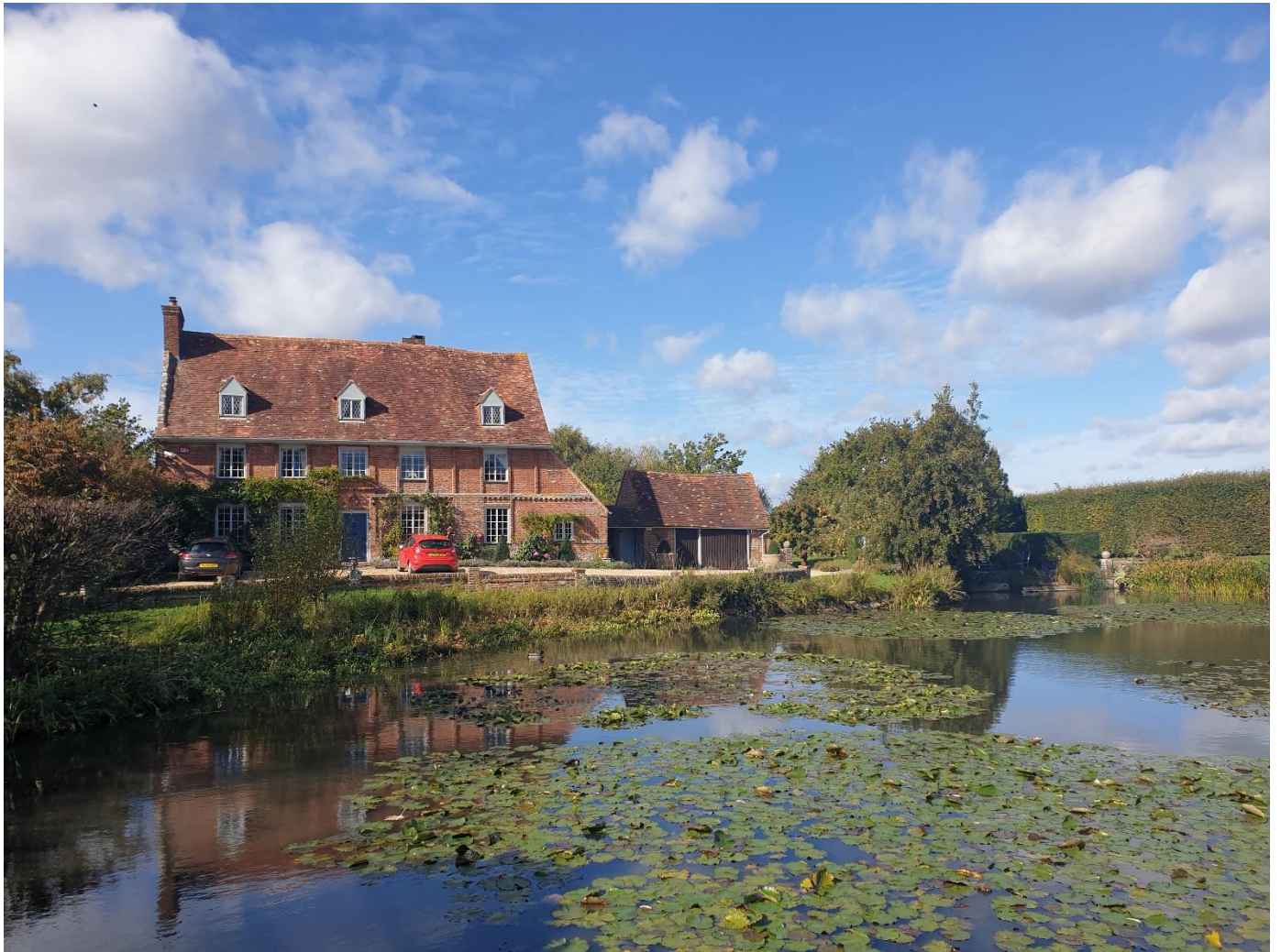
Fig 1 Front (South elevation) garage to RHS
