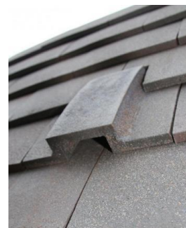
Figure 11 – Slate bat access tile.
