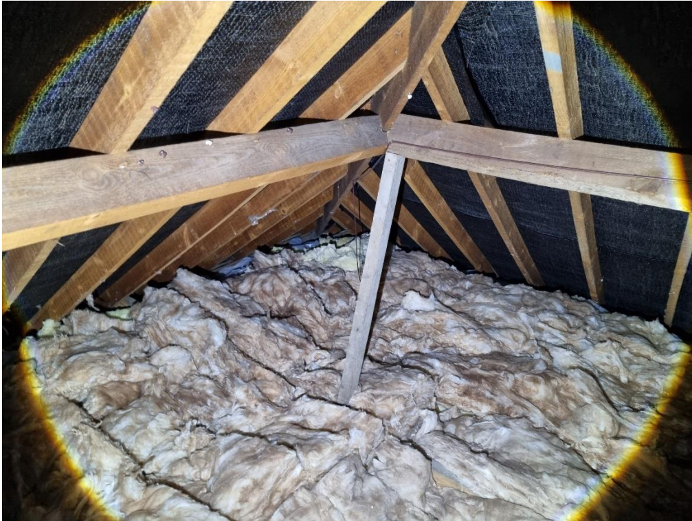
Photo 7 – Interior loft void.
