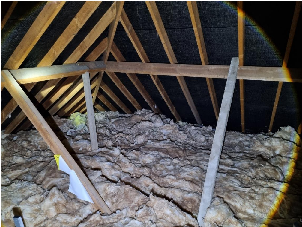
Photo 8 – Interior loft void.
