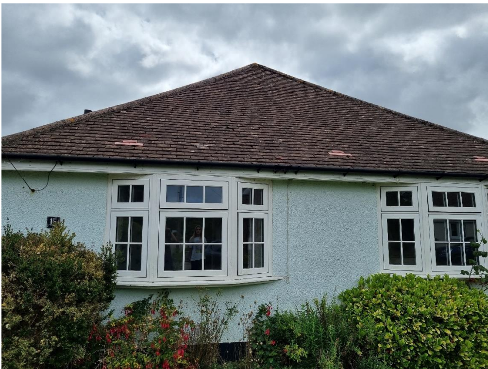
Photo 2 – West facing elevation.
