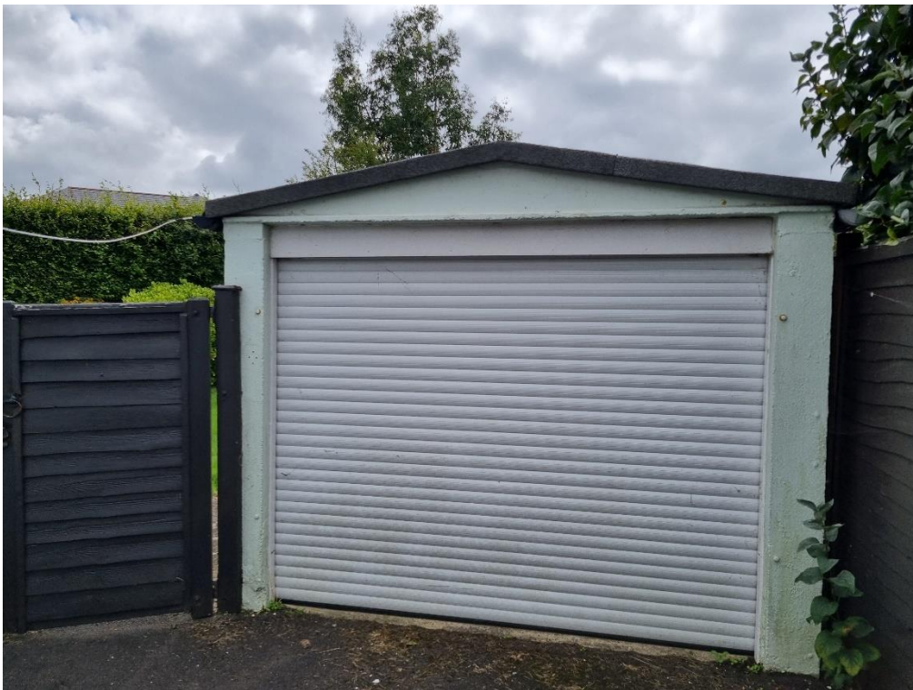
Photo 4 – West facing elevation.
