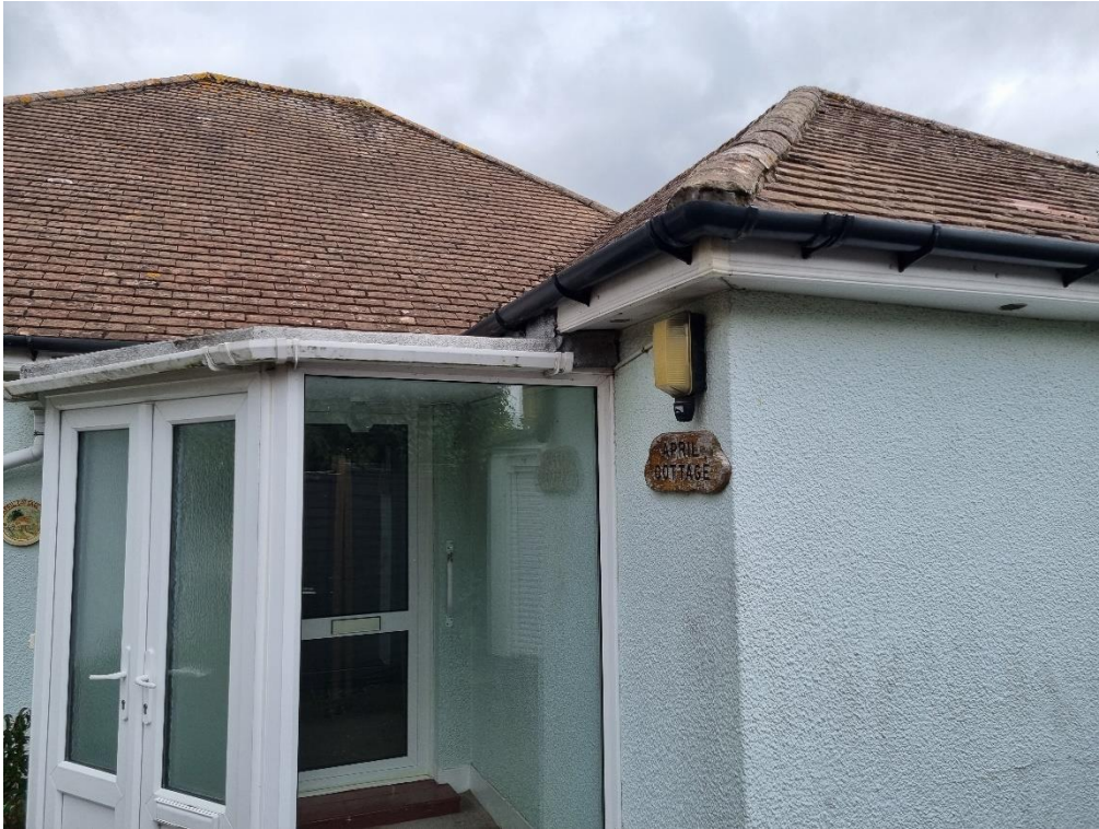
Photo 3 – South facing elevation.
