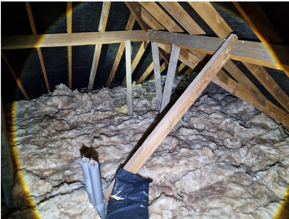
Photo 6 – Interior loft void.
