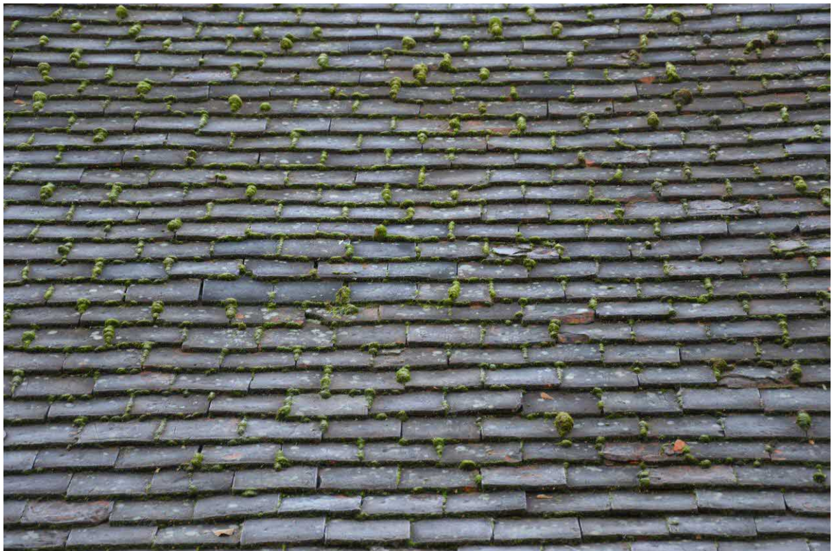
Plate 2. Tightly fitted tiles where a skylight will be installed.
