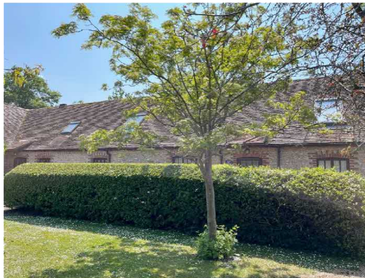
No 4 North elevation looking south
