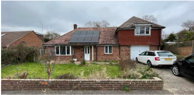
Front elevation from the kerb
