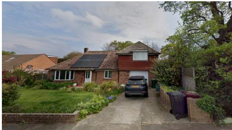
Front elevation from the kerb
