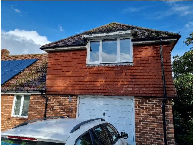
Photo 1: South facing elevation
