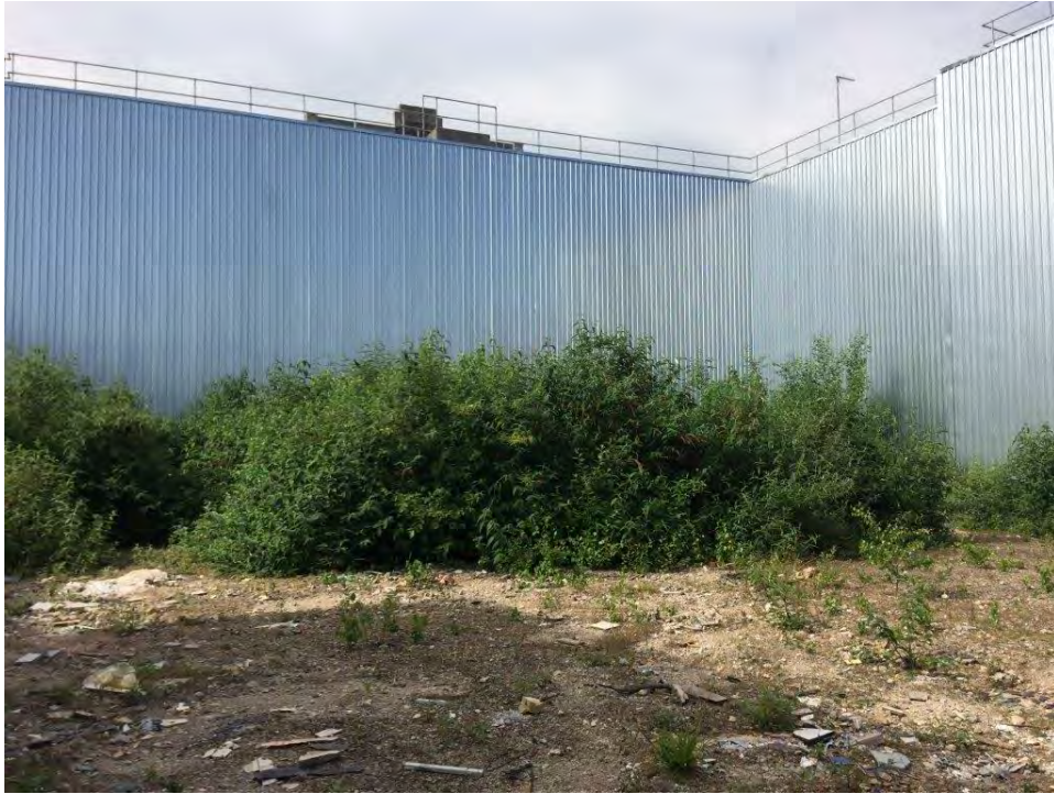
Photograph 3: Protection of retained facia on Spital Street
