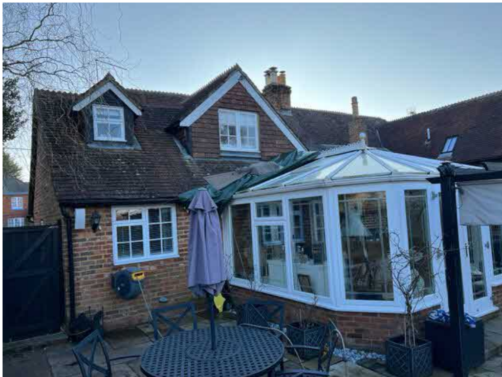
Above: Conservatory to the rear
