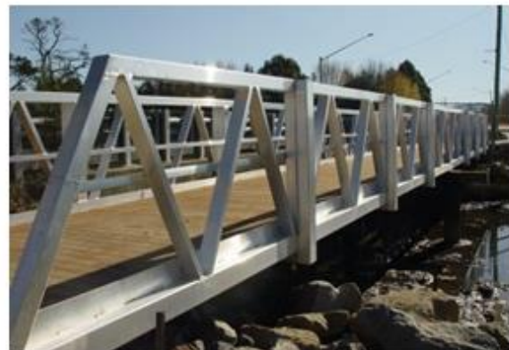
Example of Link Bridge
