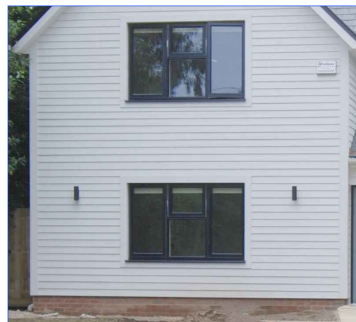
Horizontal weatherboard to rear and side elevations above brickwork
