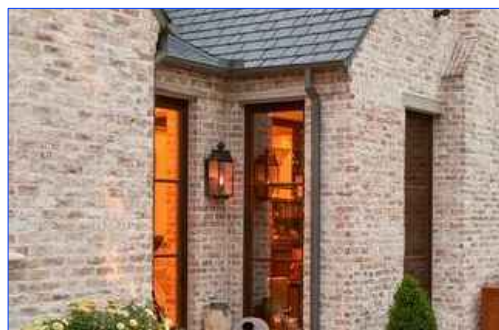
Ground floor facade in facing brickwork
