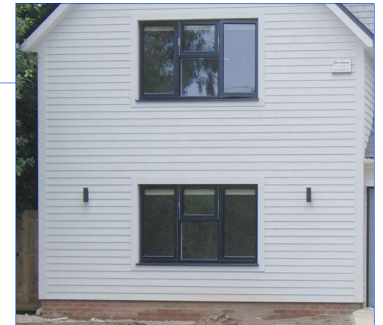
Horizontal weatherboard to rear and side elevations above brickwork
