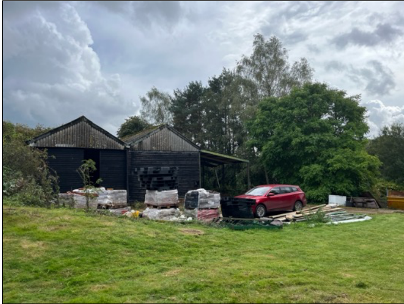
Photograph 1. A view of the managed grass on the western side of the barn.
