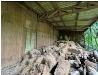
Photograph 5. A view of the plywood along the southern elevation.
