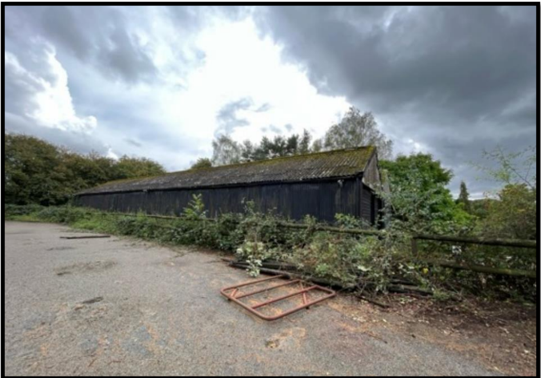
Photos of existing building
