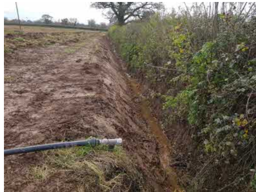
Photo 4: Recently dug drainage ditch located along hedgerow to the outer eastern boundary
