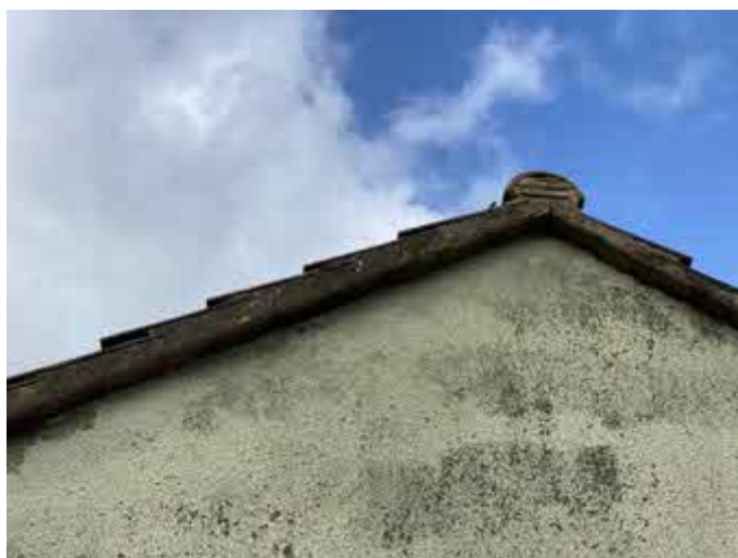
Photograph 10: Well sealed verges on the main roof.
