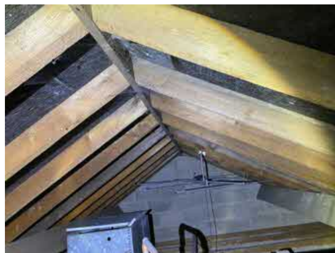
Photograph 6: Main house roof space.
