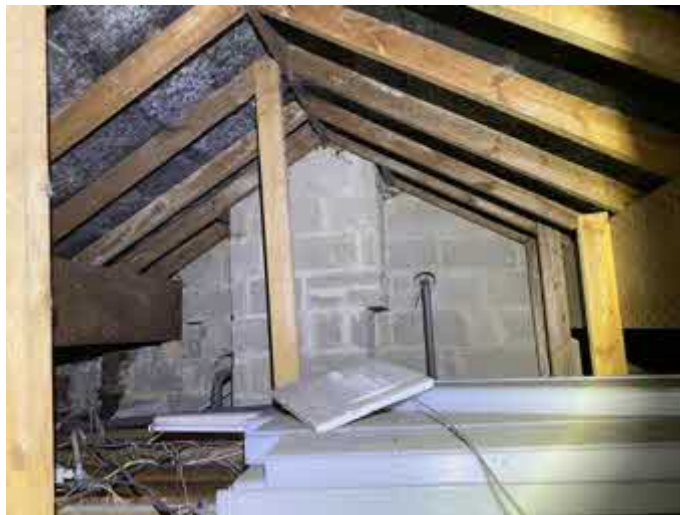
Photograph 8: Single storey section roof space.
