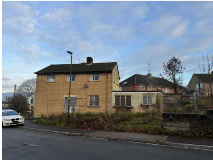
Photograph 2a: South elevation (2023).
