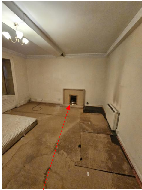
Figure 4 – Sitting Room fireplace to be removed
