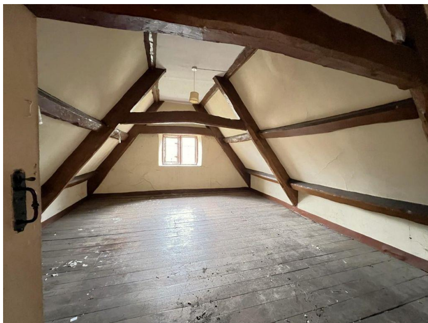
Figure 3 – Bedroom 4 where the new en-suite will be installed
