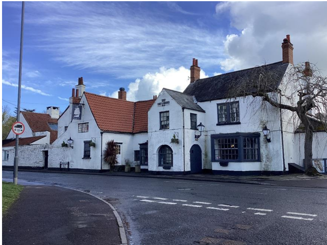
Figure 6-a - Northeast View of the Ship Inn
