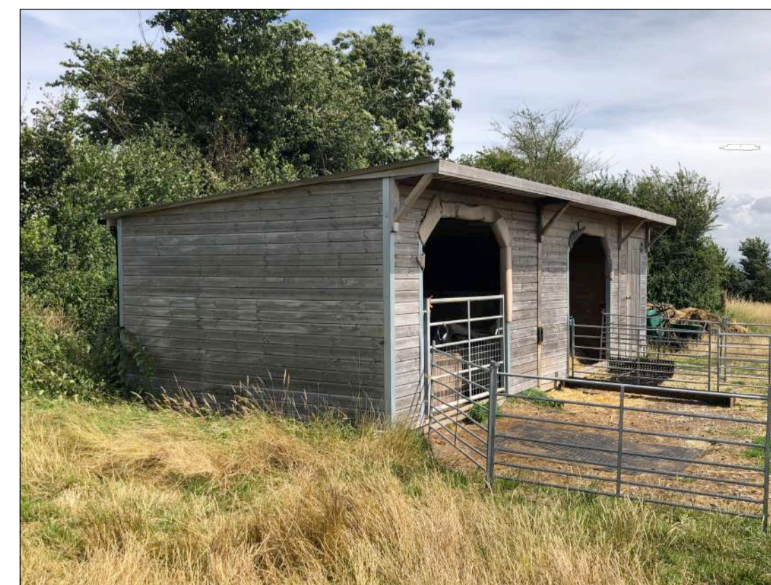
PHOTO 2: FIELD SHELTER Side
