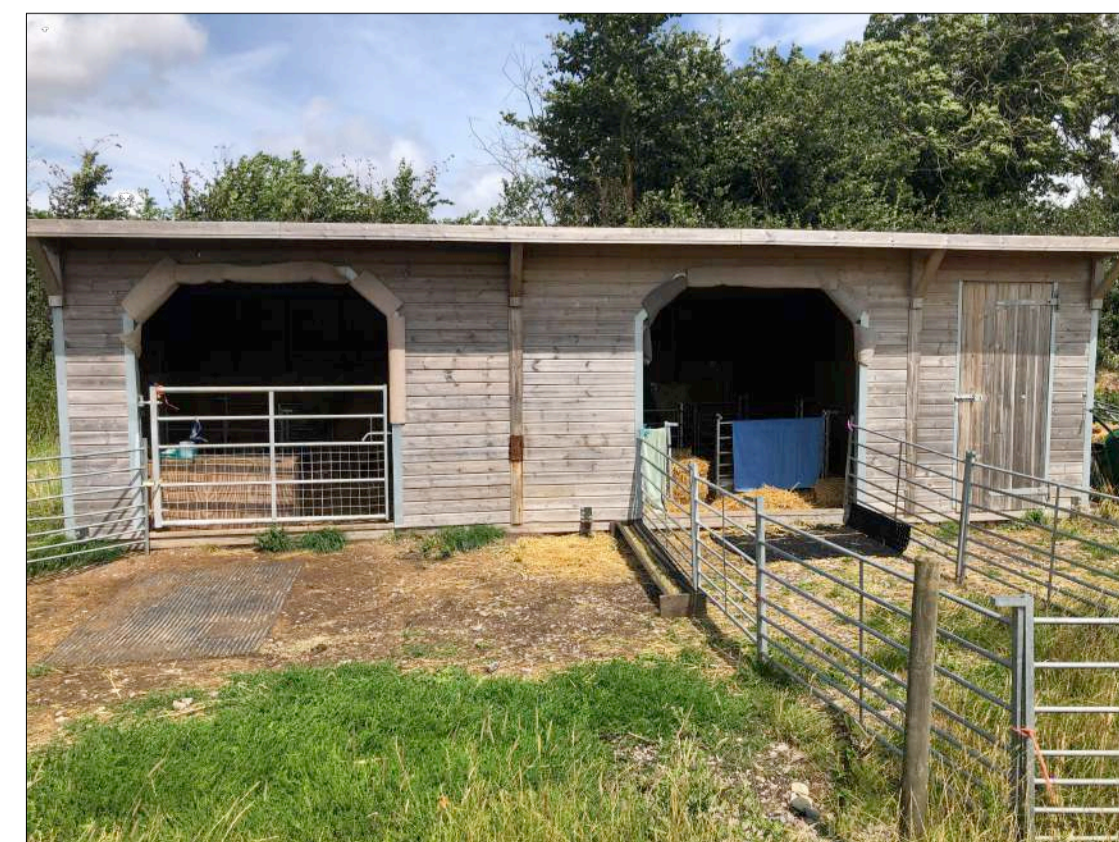
PHOTO 1: FIELD SHELTER Front
