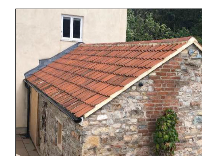
PHOTO 3: LOG STORE RE-INSTATED ROOF FINISH Existing tiles re-used, additional tiles are reclaimed tiles to match
