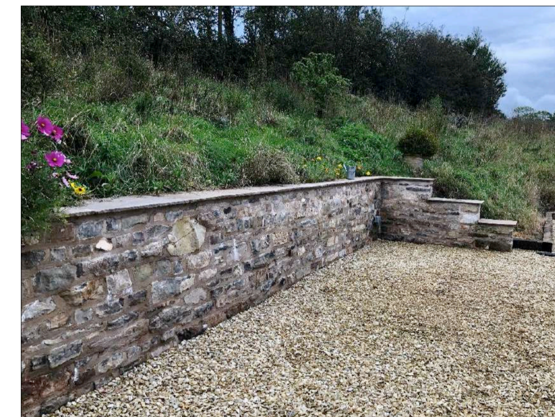
PHOTO 2: Retaining wall to back edge of terrace
