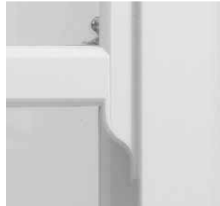
Windows with clip on sash horns (above) are not usually allowed in conservation areas whereas windows with run-through sash horns (below) have been approved.
