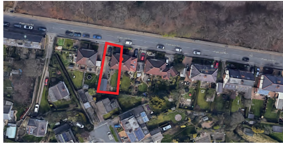
Aerial View of the property
