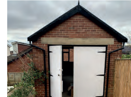
Existing Garage Entrance
