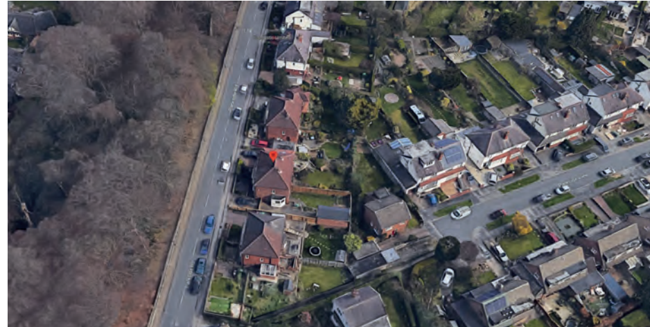
Aerial View of the property
