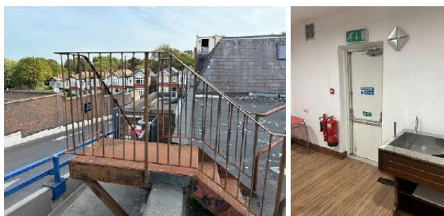
Figure 8 - Existing fire escape doors and staircase to be maintained
