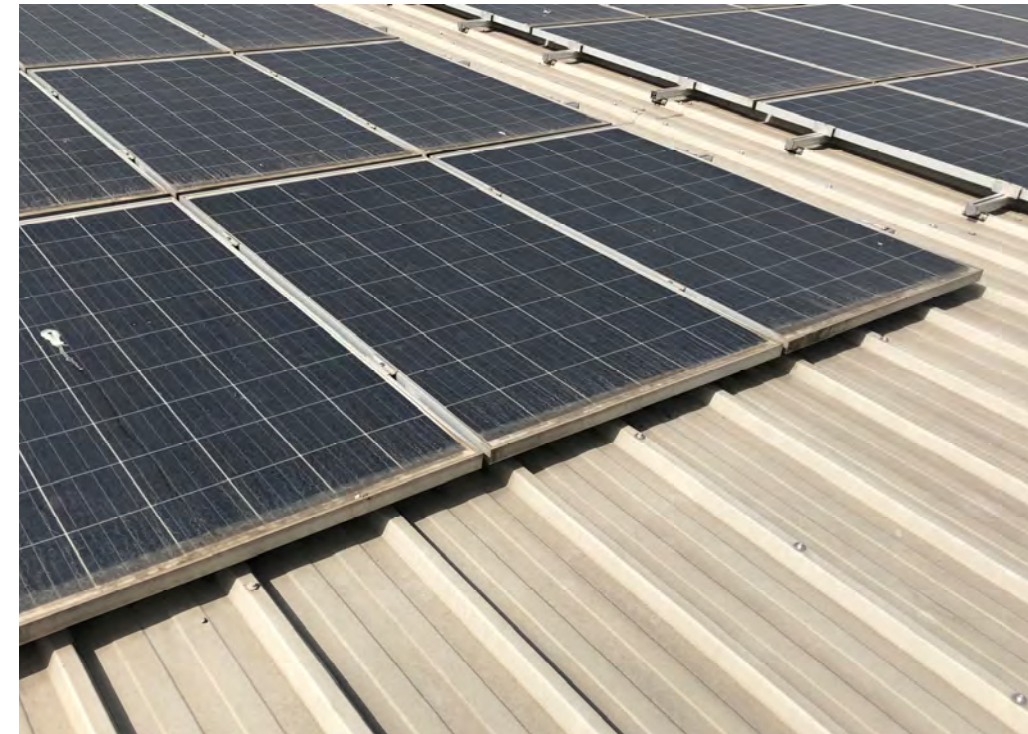
Image of roof panels with clip on photovoltaic panels
