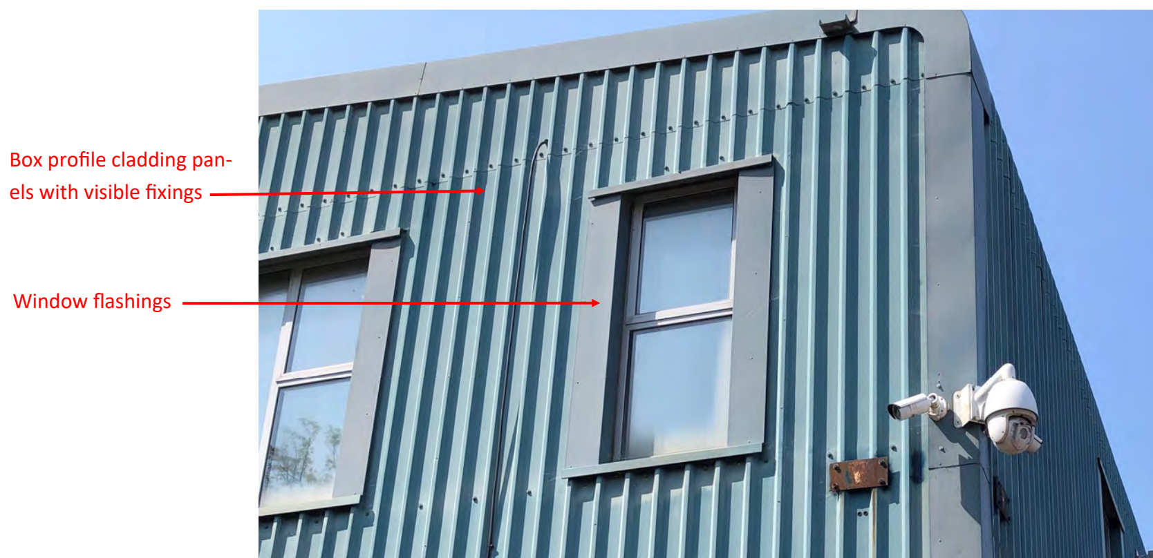
South Elevation Detail
