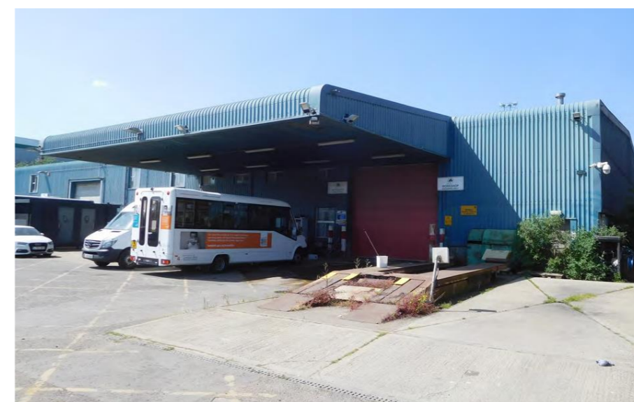
Figure 2 - Existing building exterior
