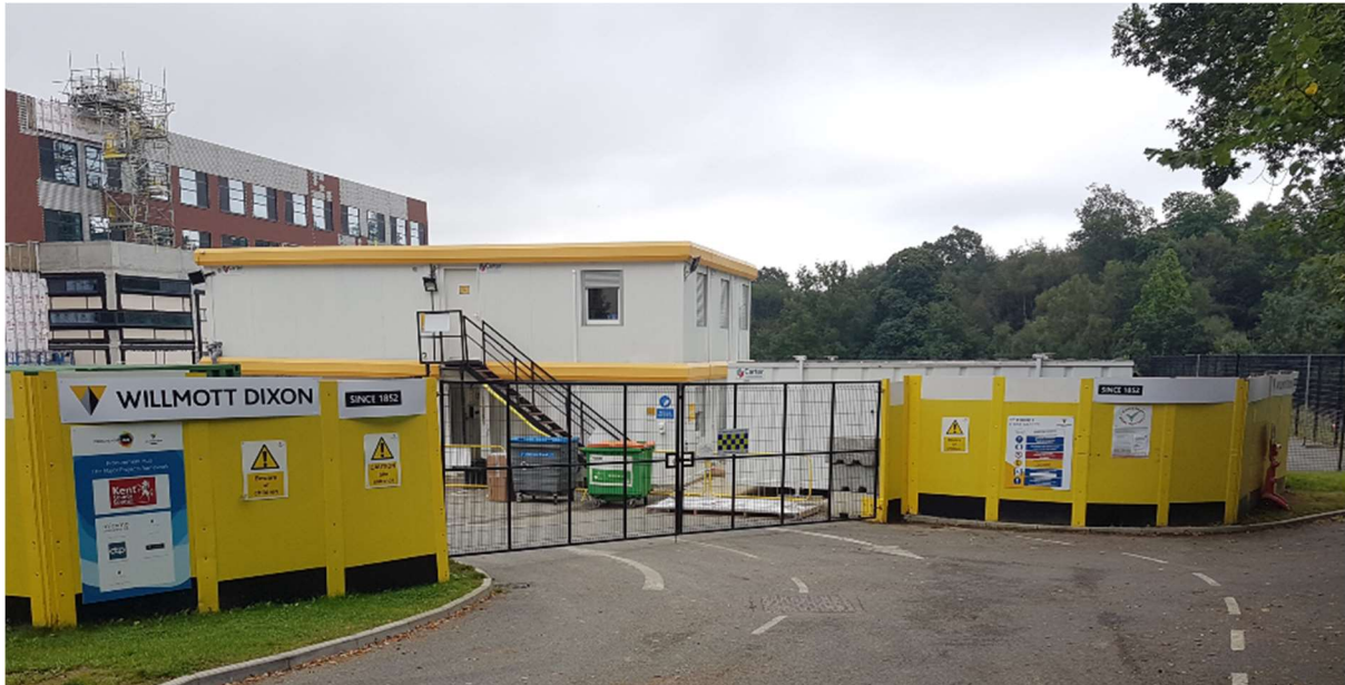
Typical Willmott Dixon site accommodation and main access gates/secure hoarding.
